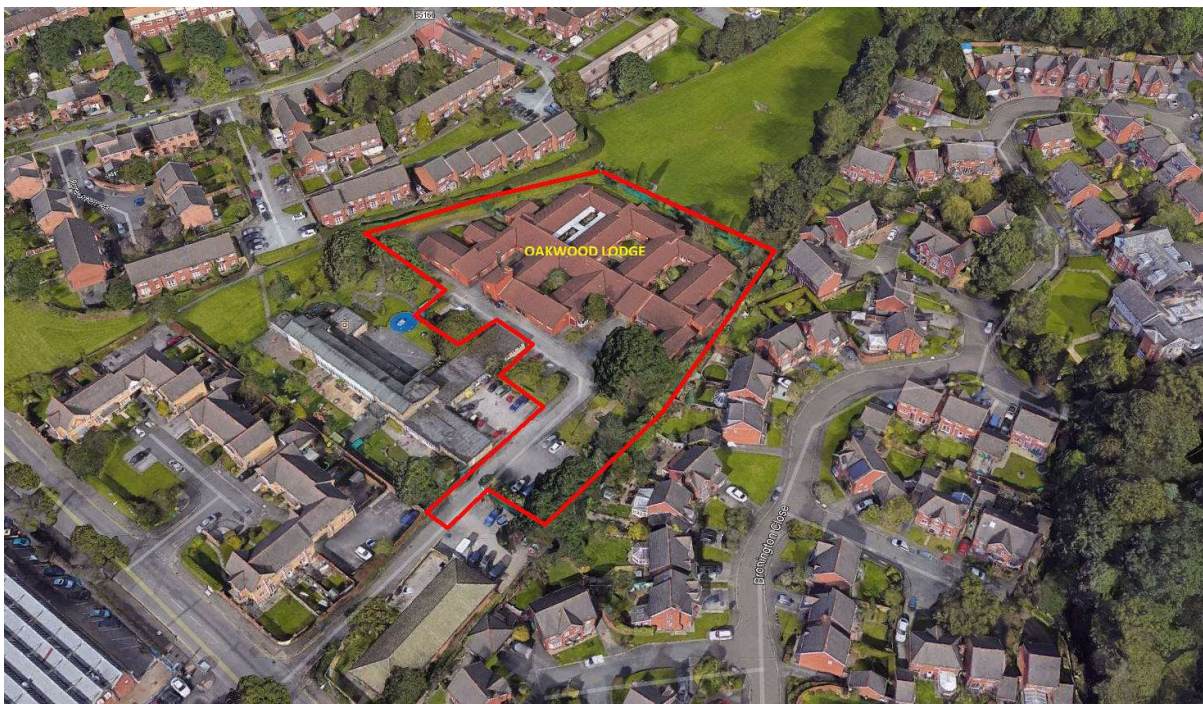
Aerial view of site, taken from Google Maps.
