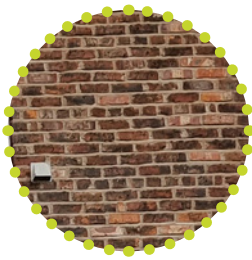
Existing red brick wall, stretcher bond
