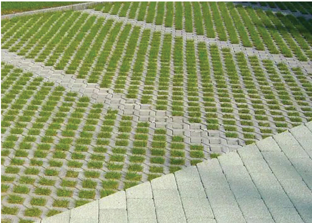
Parking: concrete grass paver blocks
