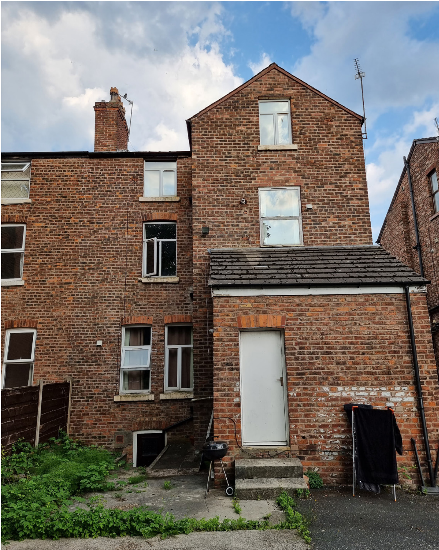
Right: The rear of 78 Clyde Road
