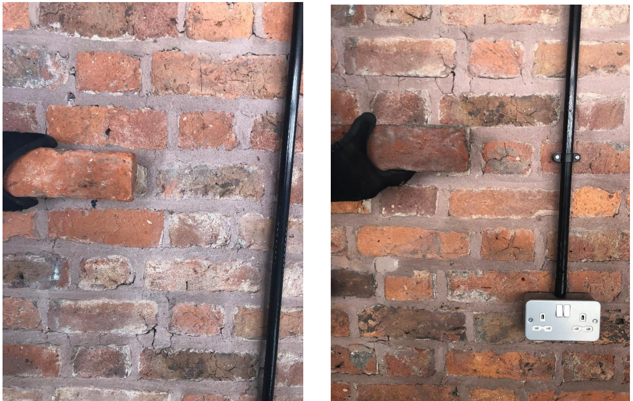
Figure 1 & 2. (above) Samples of proposed brick (sourced on site) held up against existing masonry wall.
