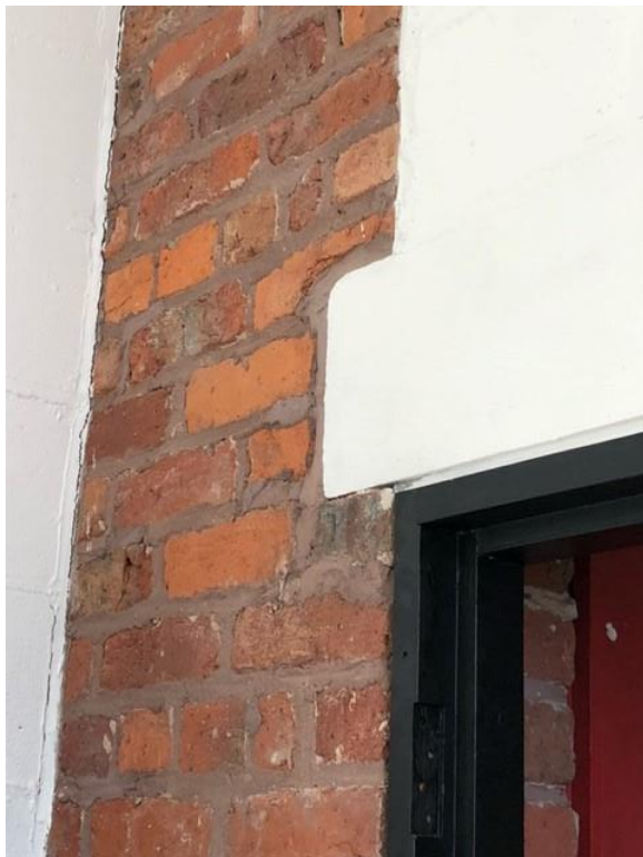
Figure 4. (left) Example of concrete lintel in existing brickwork, this is
