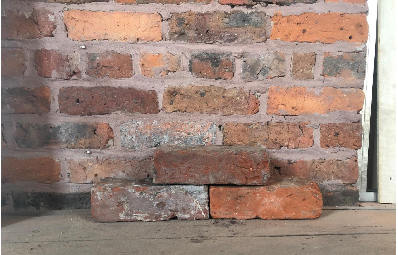
Figure 3. (above) Samples of proposed brick stacked beside existing wall.
