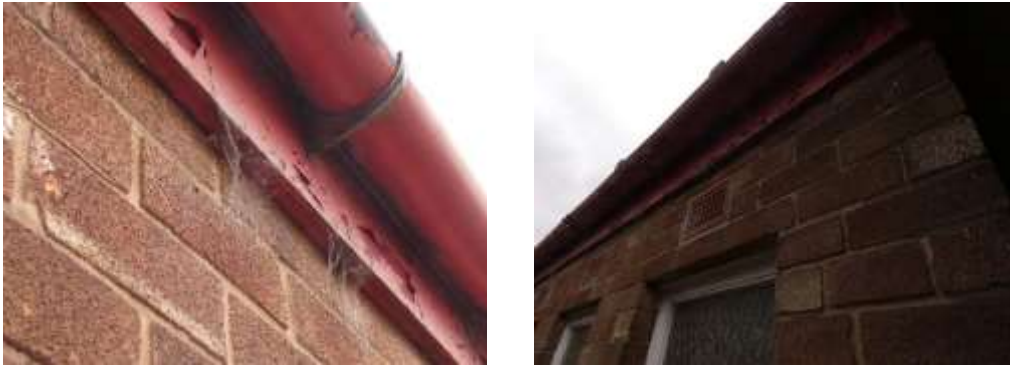
Figs. 17 & 18 Tight timber fascias
