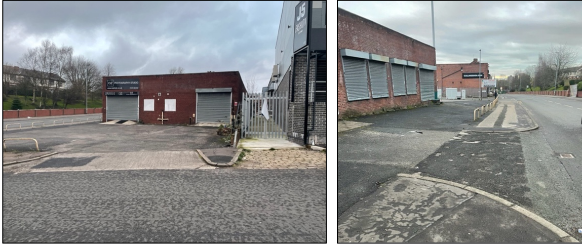
Figure 2.3: Existing accesses. Broughton Street Access (Left), Waterloo Road (Right)
