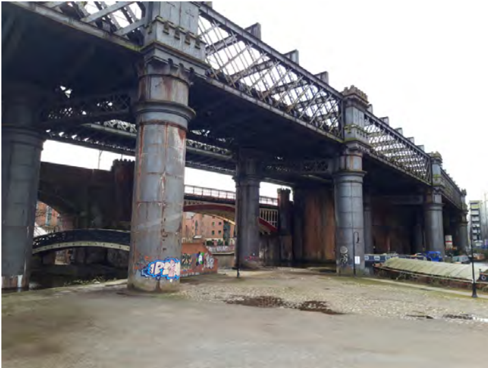
The viaduct at lower level from near Duke Street
