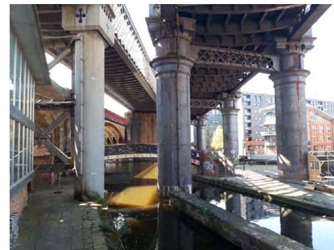
The structure crossing the Bridgewater Canal
