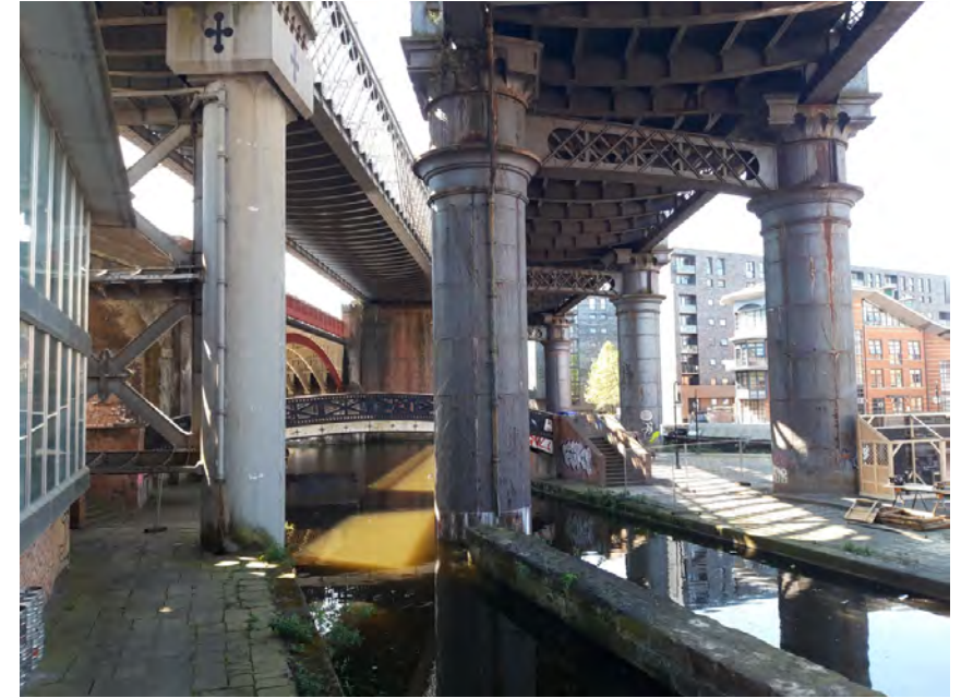
VIEW 04 From beneath the viaduct near Bar Ca looking along the structure and across the canal
