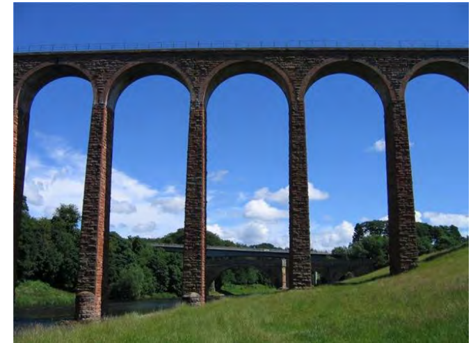
The Leaderfoot Viaduct, Scottish Borders
