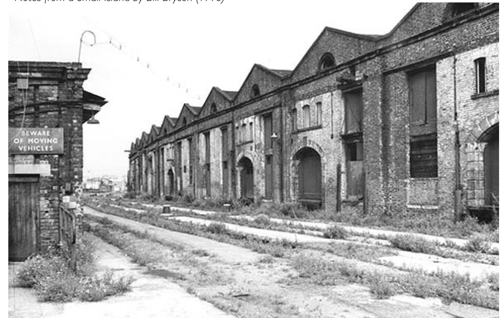
The then abandoned Liverpool Road Station in 1985
