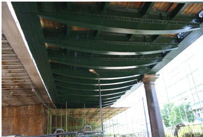
Rockingham Street Bridge, London (c. 1890s)
