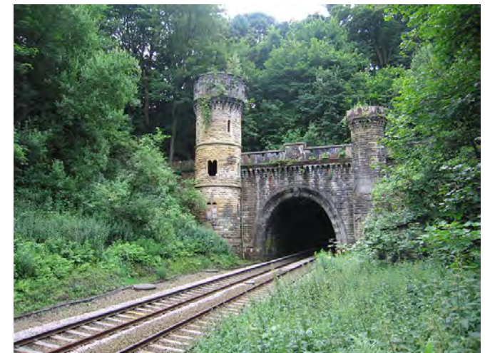
Bramhope Tunnel, West Yorkshire
