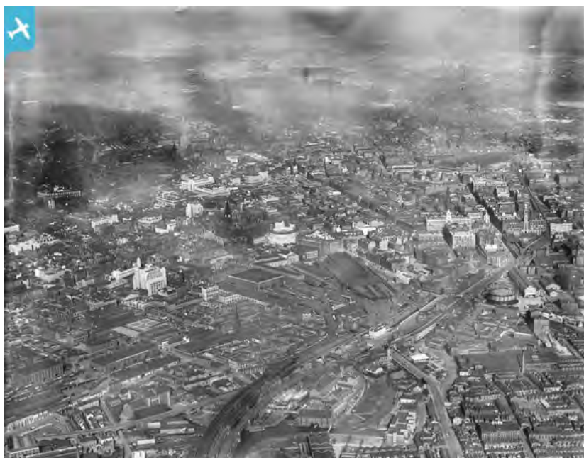
Aerial photo from 1934 showing the viaduct at the bottom of the image
