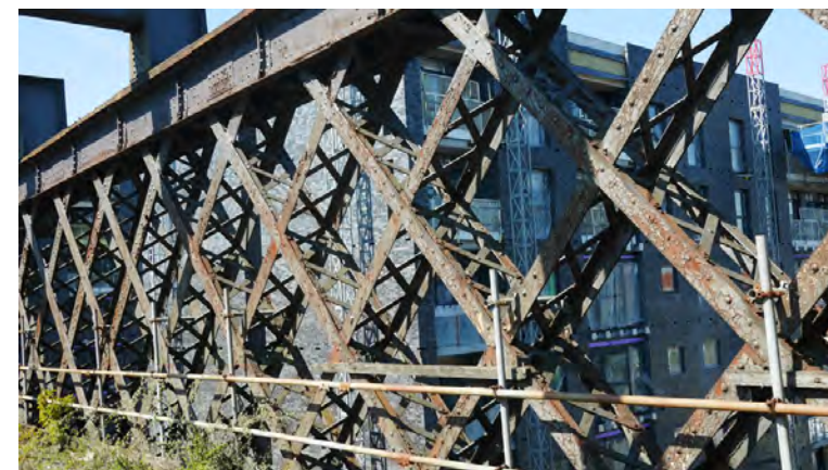
The lattice steelwork by Heenan and Froude
