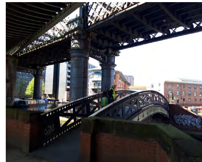
The viaduct crossing the Bridgewater Canal
