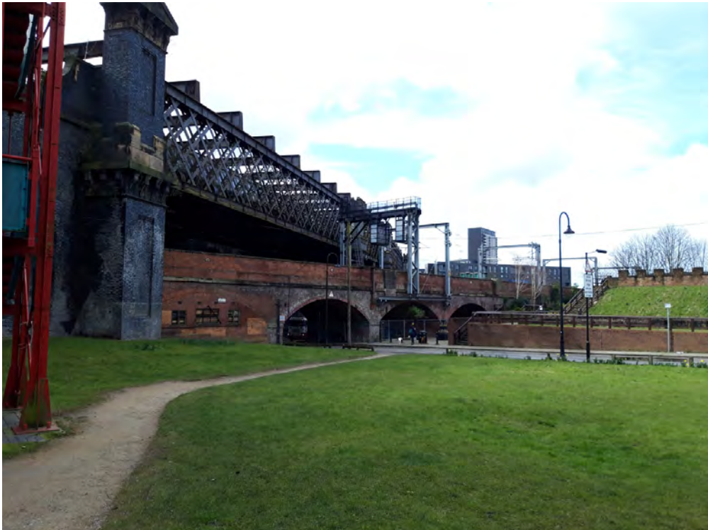
VIEW 01 From the Roman fort across the urban park
