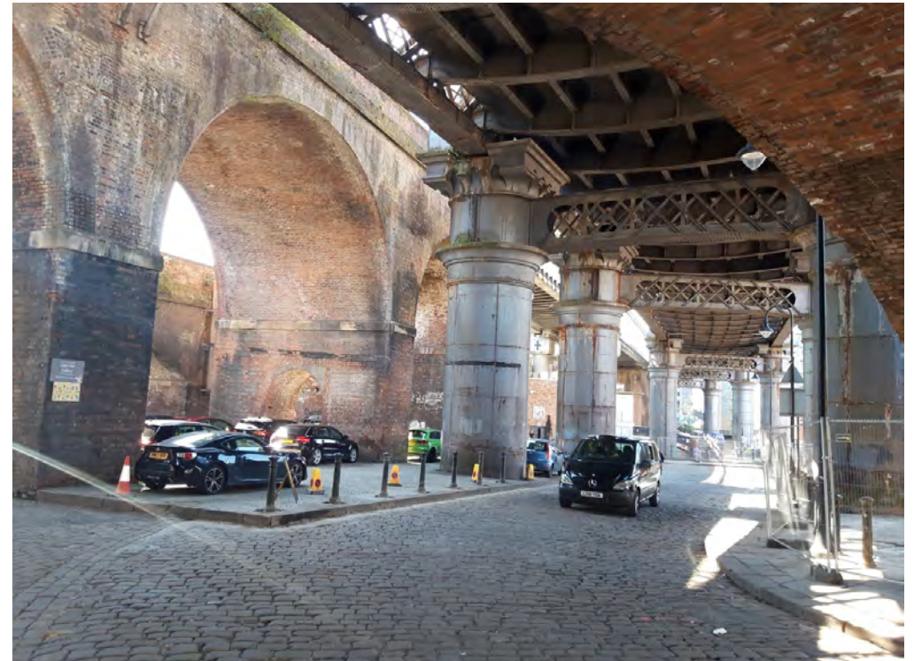
VIEW 02 From Duke Street looking along the length of the viaduct
