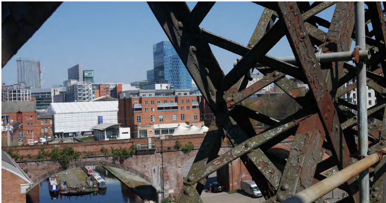
The view looking south from the viaduct across the canal basin
