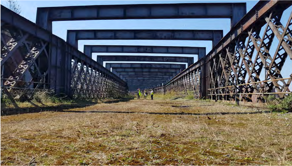
VIEW 03 From on the viaduct looking along its length
