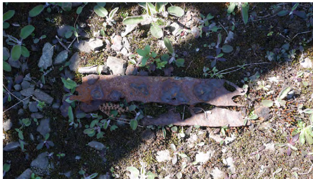
Pieces of scrap metalwork found across the structure, probably the original overhead bracing
