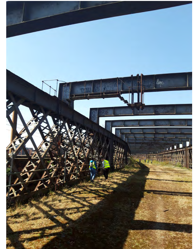
The overhead bracing and ladder access in one location
