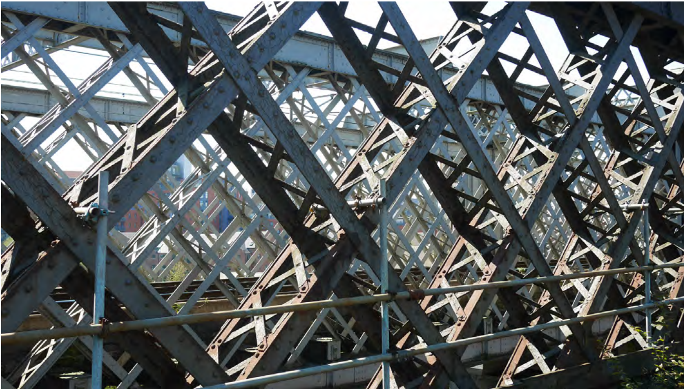
The lattice work on each side of the viaduct
