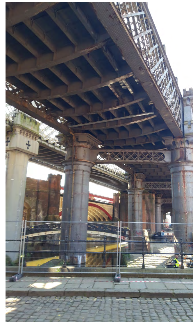
Beneath the viaduct showing the fish bellied deck
