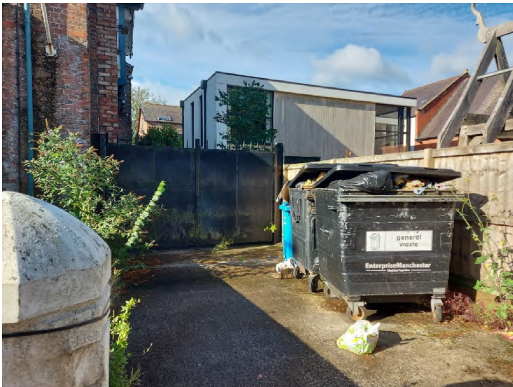
Photograph 4 - Bin Storage Area to Front of Property
