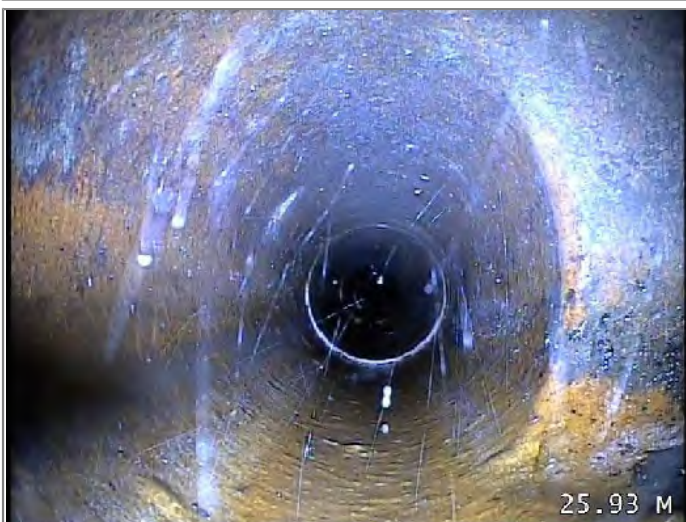
Junction at 3 o'clock, diameter 100mm
