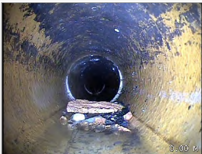
Start node type, manhole, reference MH 02
