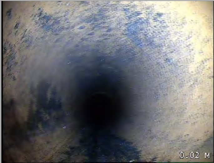
Start node type, manhole, reference MH 03
