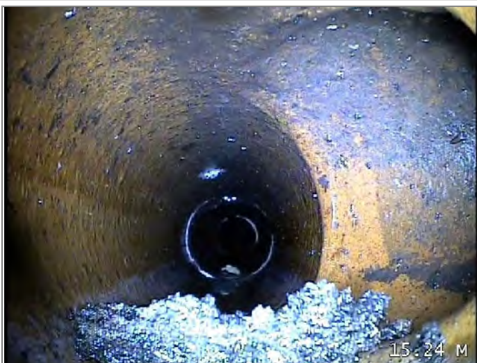
Junction at 3 o'clock, diameter 100mm
