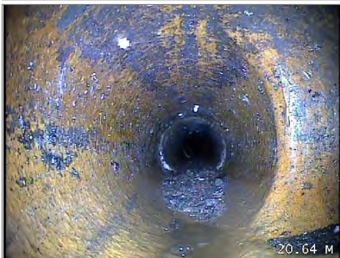
Junction at 3 o'clock, diameter 100mm
