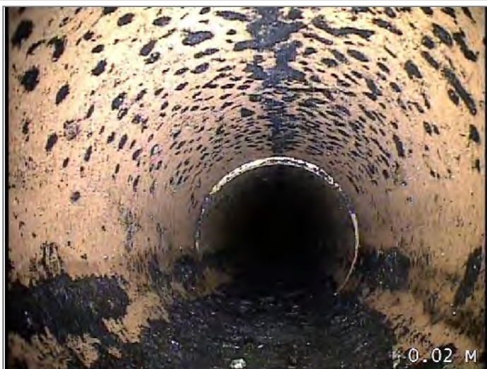
Start node type, manhole, reference MH 03
