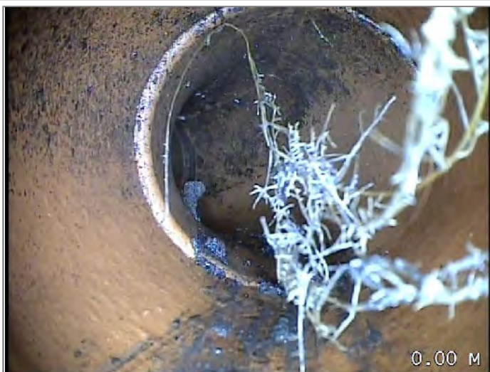
Start node type, manhole, reference MH 02
