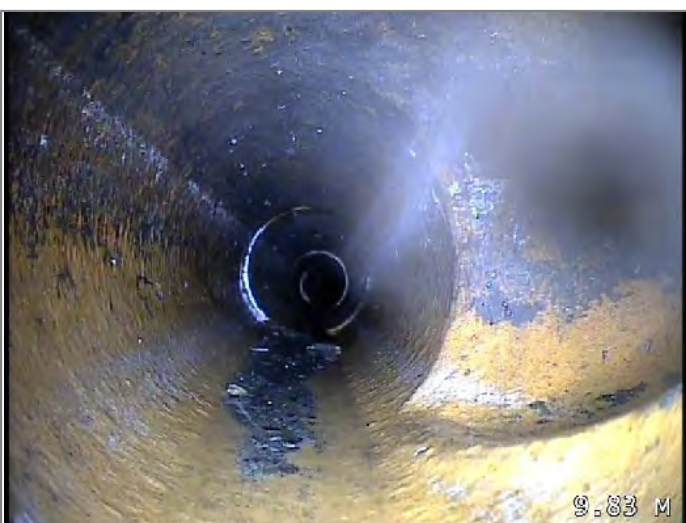
Junction at 3 o'clock, diameter 100mm
