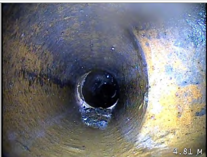
Junction at 3 o'clock, diameter 100mm
