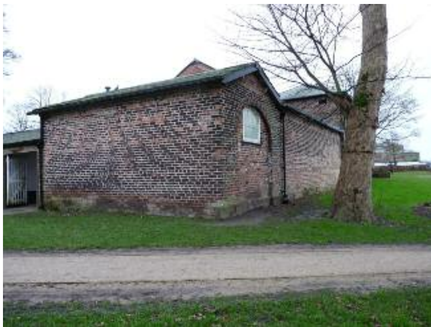
Fig.13: south-west corner of the stable complex
