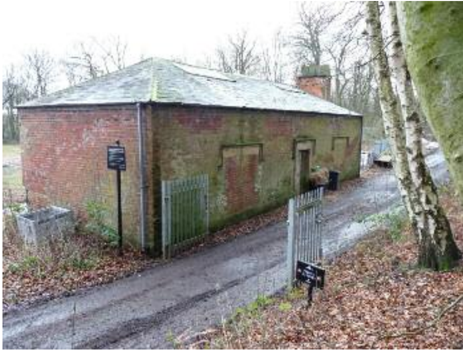
Fig.27: the 'dairy' from the north-east
