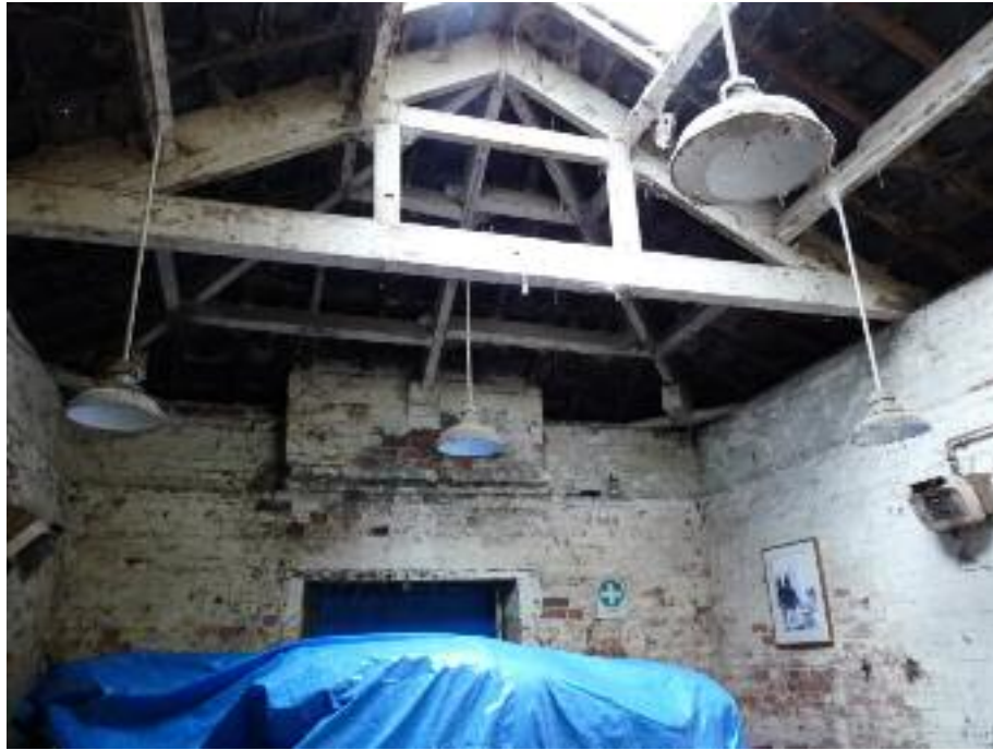
Fig.29: interior of 'dairy' from the east, in the west room
