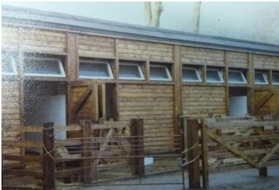
Fig.14: undated photograph from the 1980s showing newly built animal boxes in the west range (Heaton Park Animal Centre archive)
