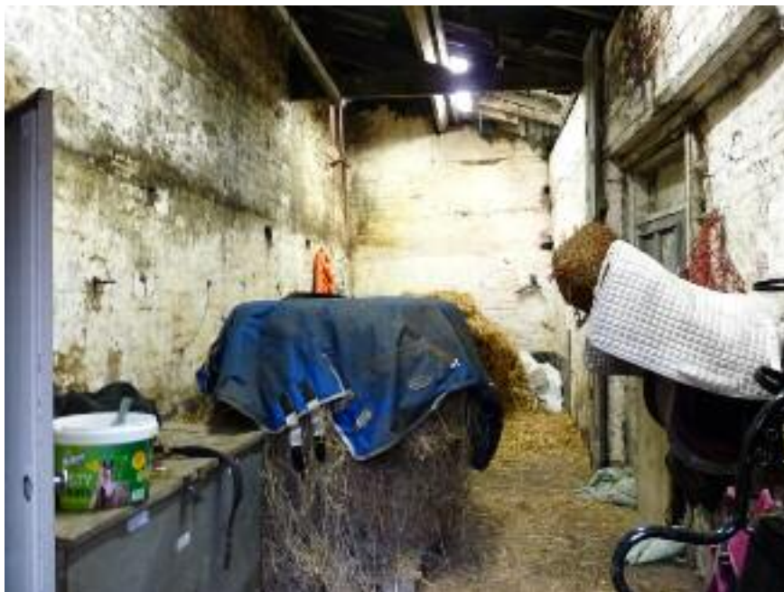
Fig.34: internal view of east backshed, from the east
