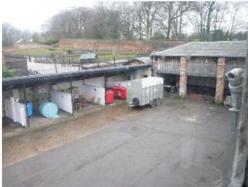
Fig.20: the west and north sides of stable yard, from first floor over through passage
