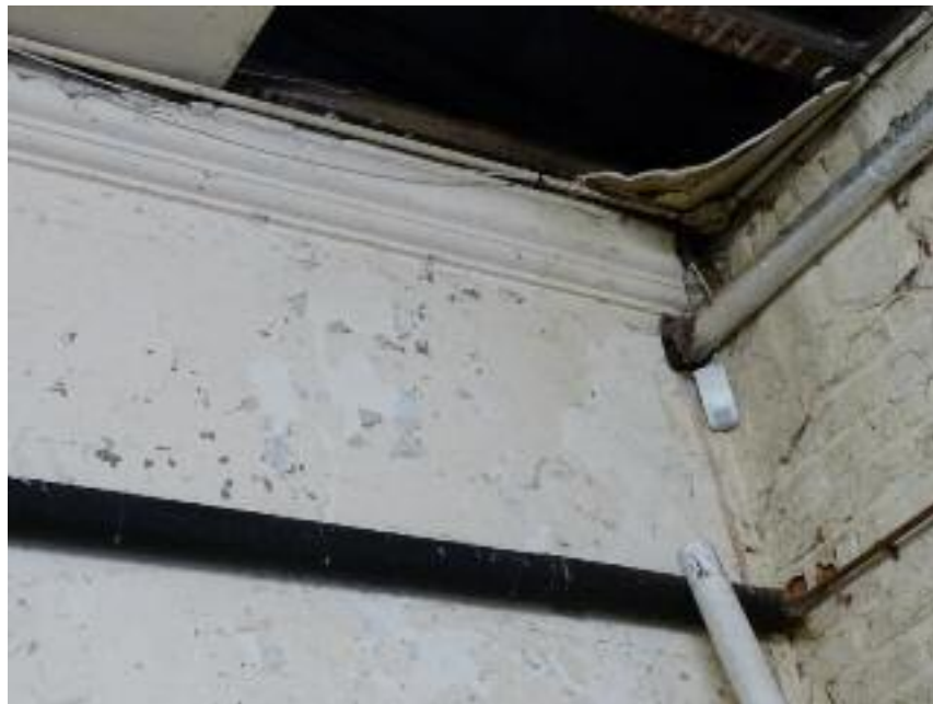
Fig.11: fragment of plaster cornice in the north stable (south wall)
