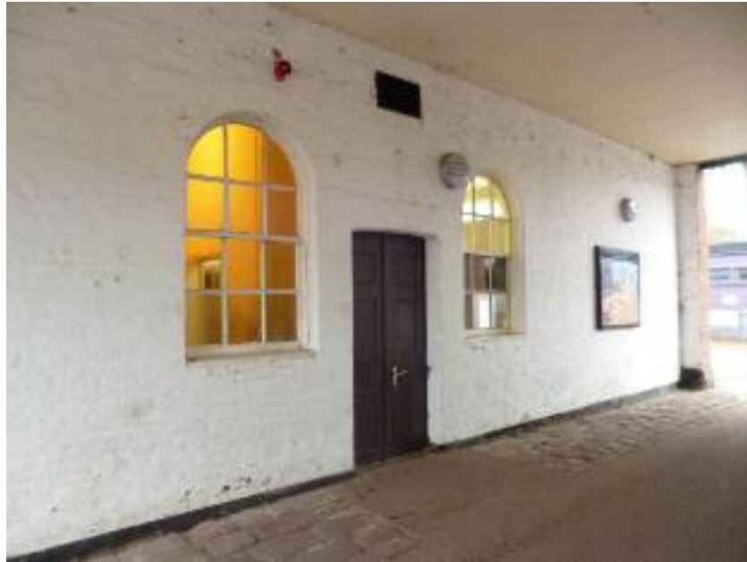
Fig.8: north side of through passage with original central doors and sash windows to harness room
