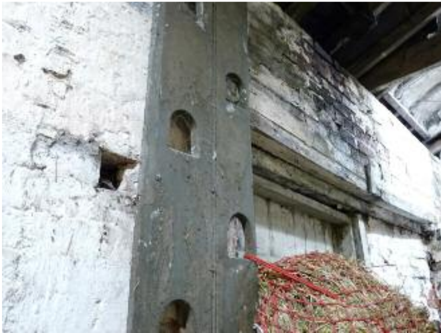
Fig.35: ladder to former loft in east backshed
