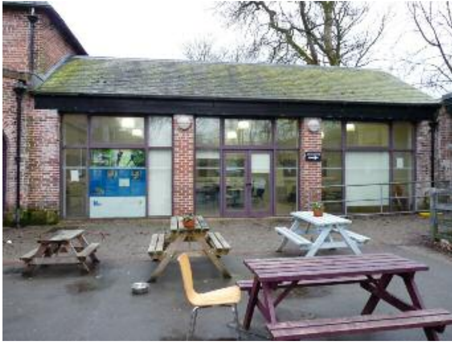
Fig.21: south range to yard, refurbished in 2003-04 for a learning centre
