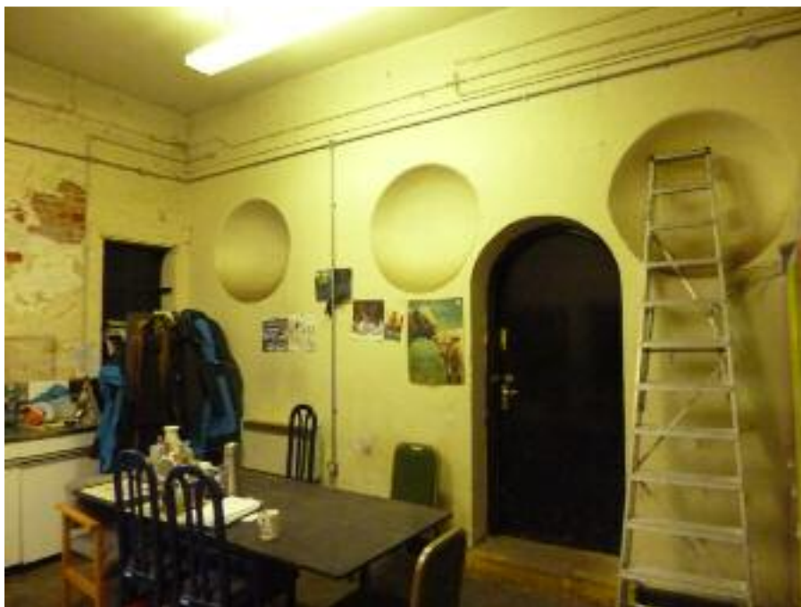
Fig.17: Former 3-stall stable in north pavilion, probably for coach horses (arched doorway is later)
