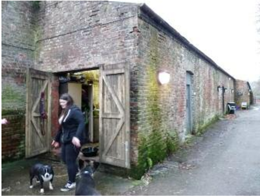
Fig.31: the backsheds from the east
