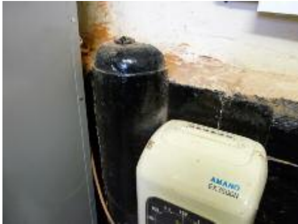
Fig.9: stall post and timber wall lining on south wall in north coach house
