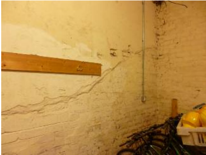
Fig.16: ghost curved profile of wall lining to a removed stall in the north stable
