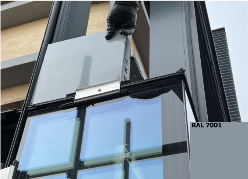
Adjusted photograph of 7001 gloss panel at the head of the lift shaft
