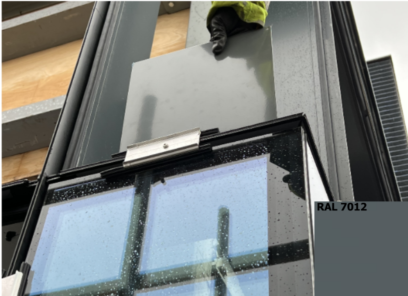
Photograph of 7012 gloss panel at the head of the lift shaft
