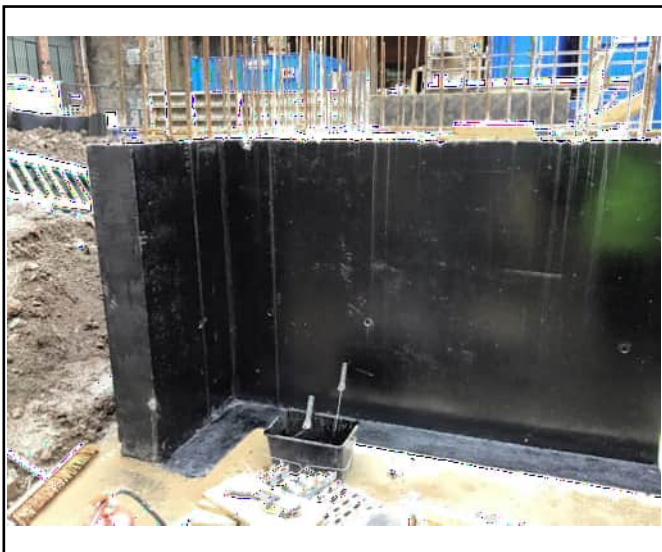
Primed wall with bucket of primer
