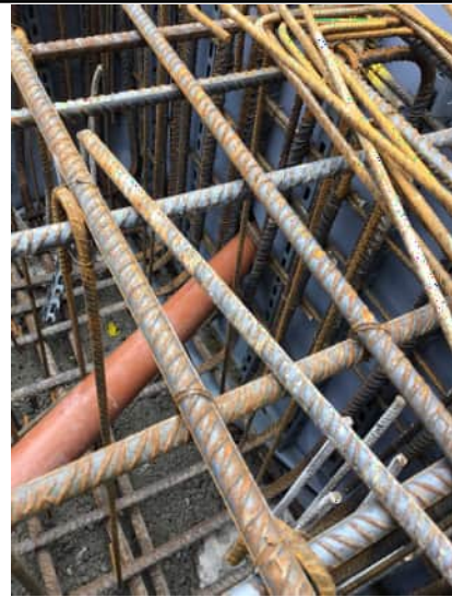
Internal section of pipe within pile cap
