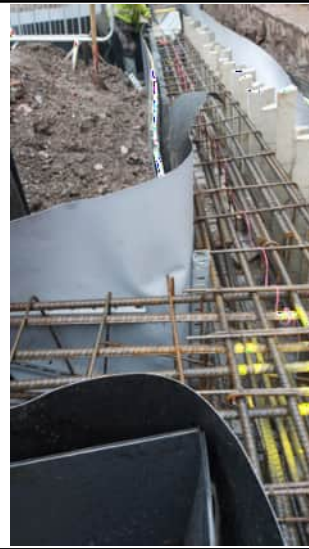
Overview of ring beam with visqueen
