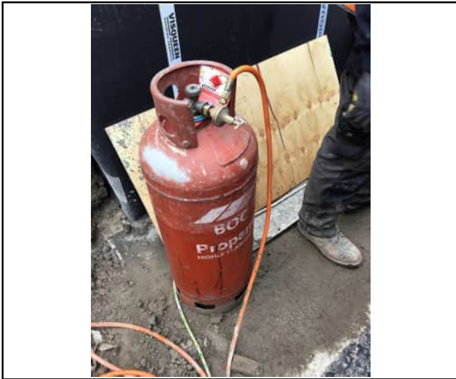
Gas used to prime bitumen
