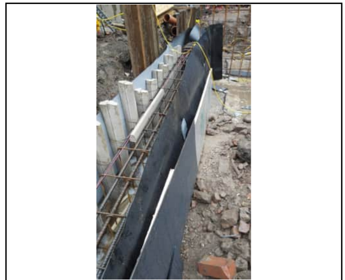
Ring beam showing wrapped membrane
