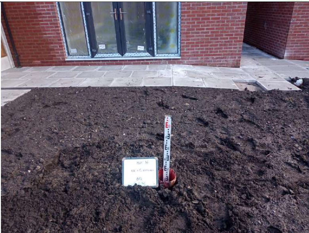
Photograph 2: Validation of Garden Capping Thickness
