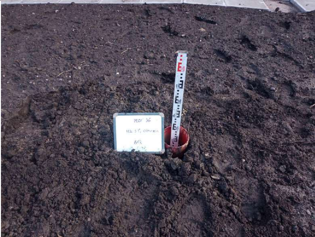
Photograph 1: Validation of Garden Capping Thickness
