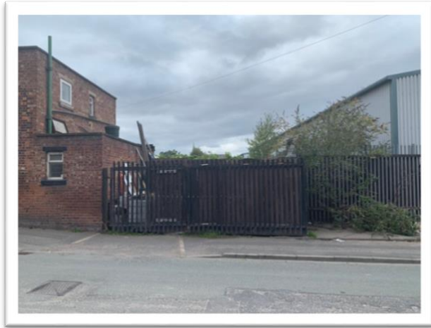
View to site entrance
