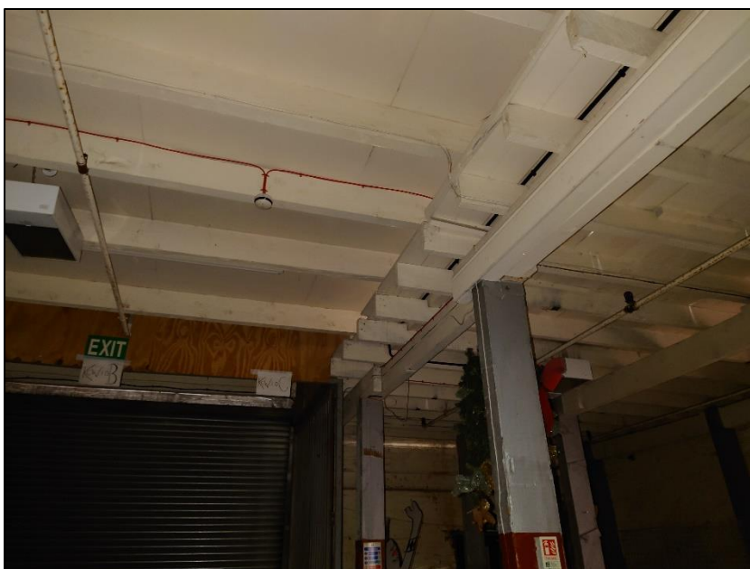
Photograph 8 showing the interior ground floor of the warehouse area
