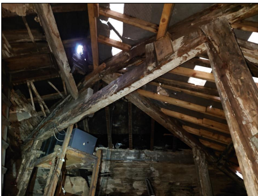
Photograph 12 showing the roof void of the former public house
