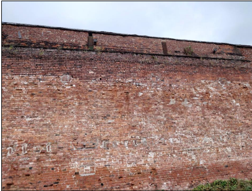
Photograph 2 showing the brickwork
