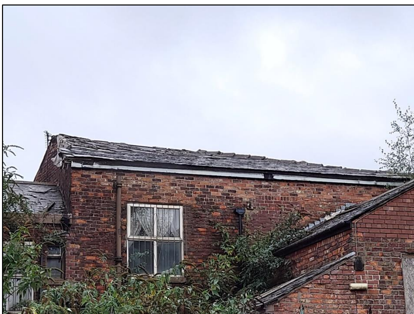
Photograph 10 showing the roof of the former public house
