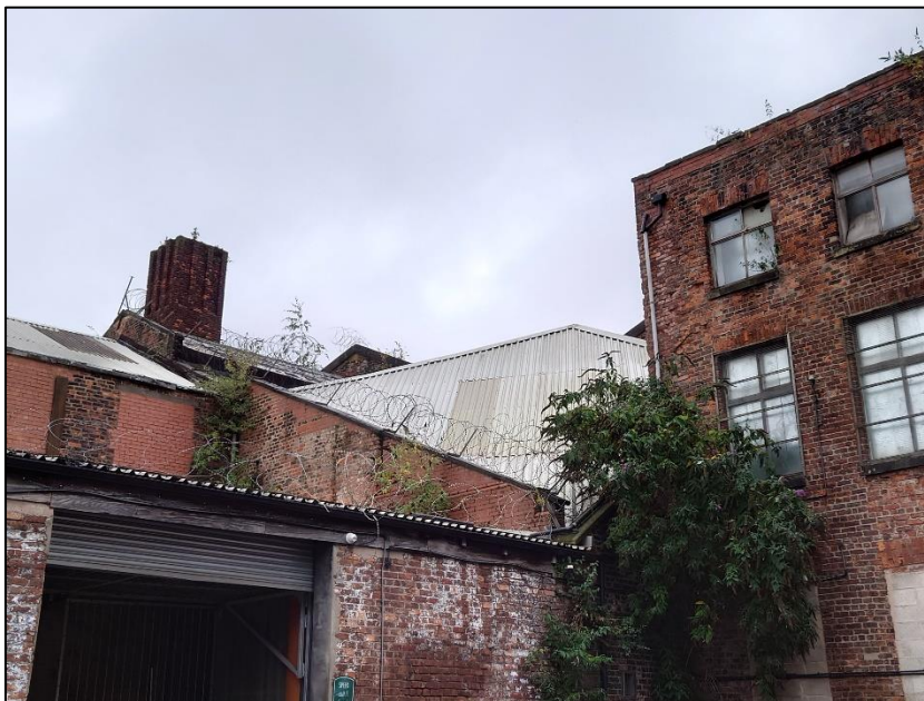
Photograph 5 showing the roof of the upper floor
