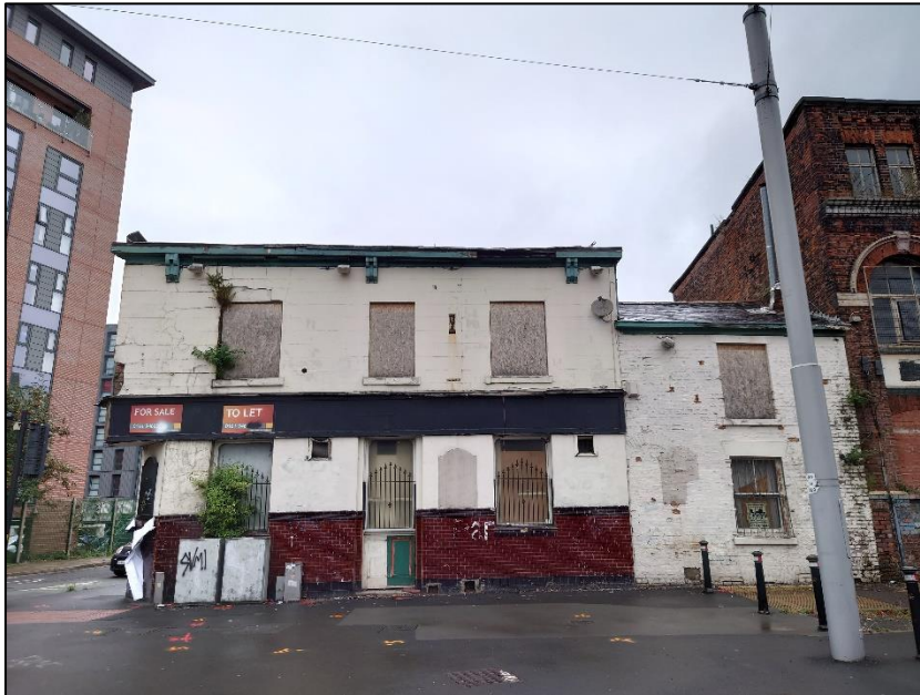
Photograph 9 showing the exterior of the former public house
