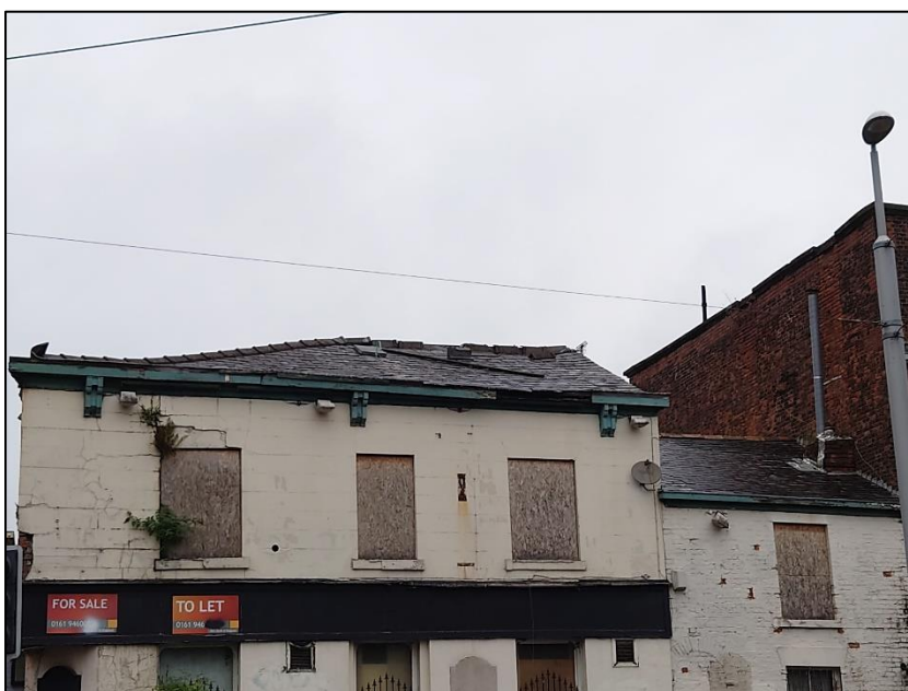
Photograph 11 showing the roof of the former public house
