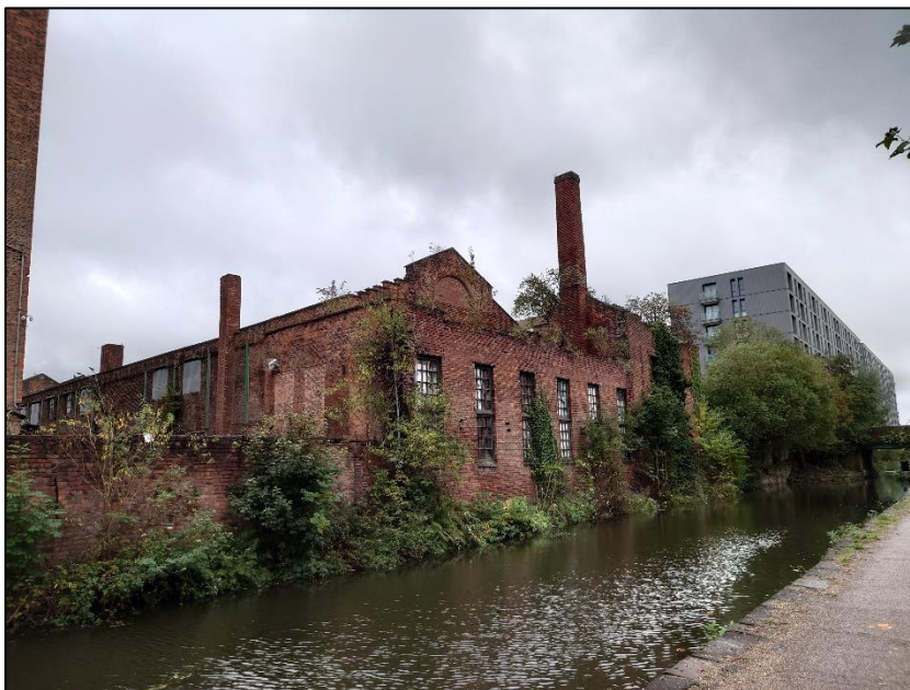
Photograph 3 showing the exterior of the building from the canal towpath
