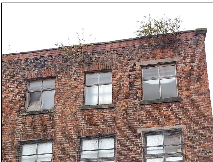
Photograph 1 showing the external brickwork
