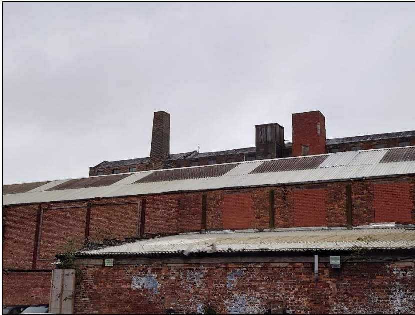
Photograph 4 showing the roof of the warehouses
