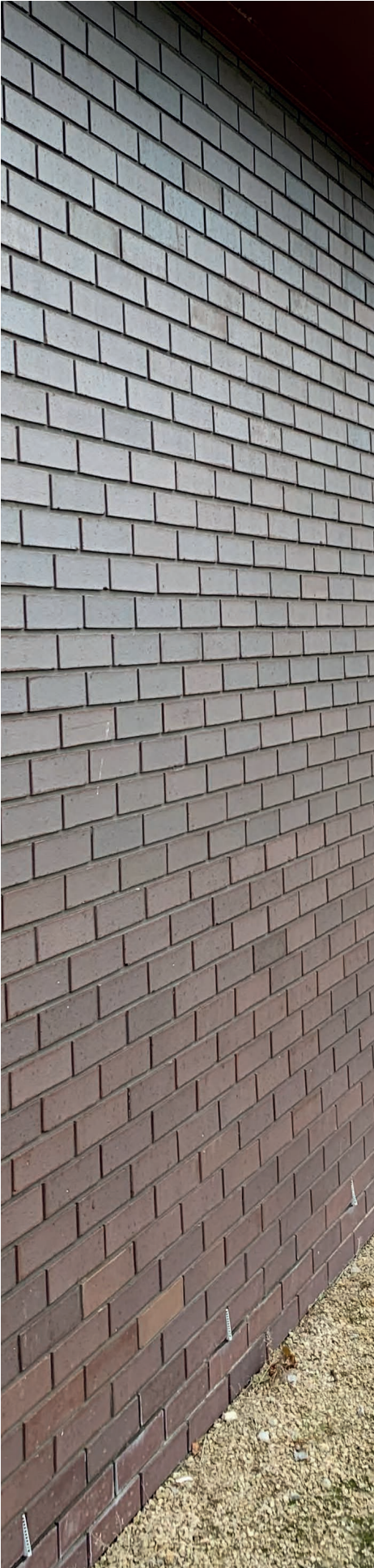
Brickwork To match the existing building
