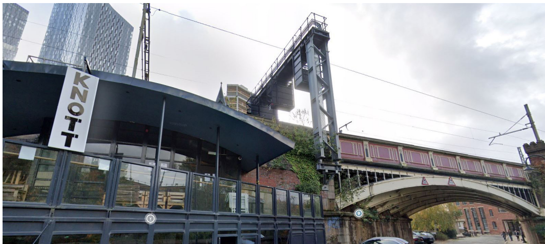
Figure 6 Signal 3- located outside Deansgate Station on track 6 westbound
