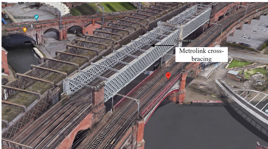
Figure 17 Metrolink (Track 3 and 4) cross-bracing structure
