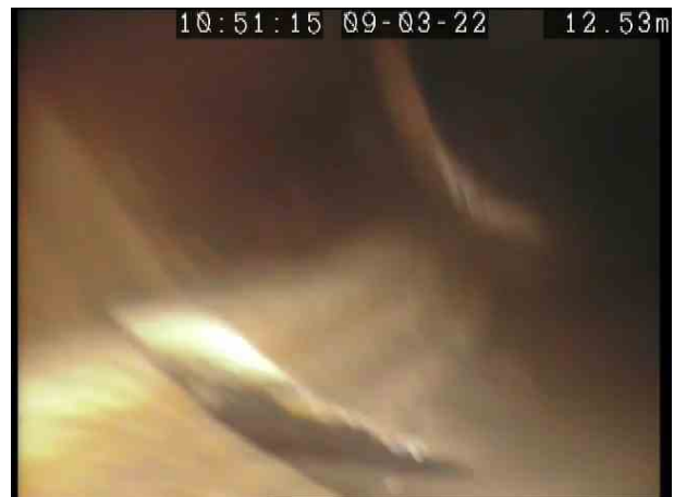
USX_ac4bbd2e-af05-4421-b905-e751a3f9c9b1_20220321_162010_813.jpg, 00:01:31, 12.53 m Open joint, large
