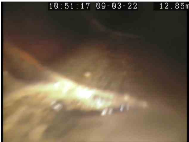
USX_53b274df-1a01-43b9-b3e5-40efbcdace4f_20220321_162219_102.jpg, 00:01:32, 12.85 m Joint displaced, medium
