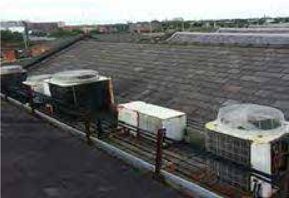
Existing M&E Plant to be removed from roof valley of Bay05. Extract from 261 Design and Access Statement Page 10. Updated Feb 2020.
