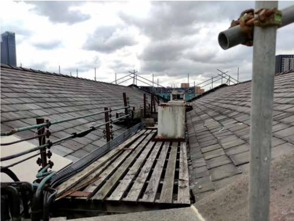
Existing M&E Plant to be removed from roof valley of Bay05. Photo from scaffold June 2021.
