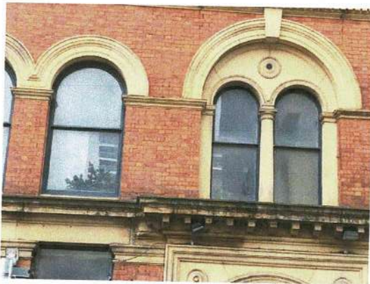
Typical sash windows for redecoration.
