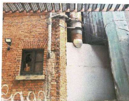
Remove cement parging and replace SVP.
