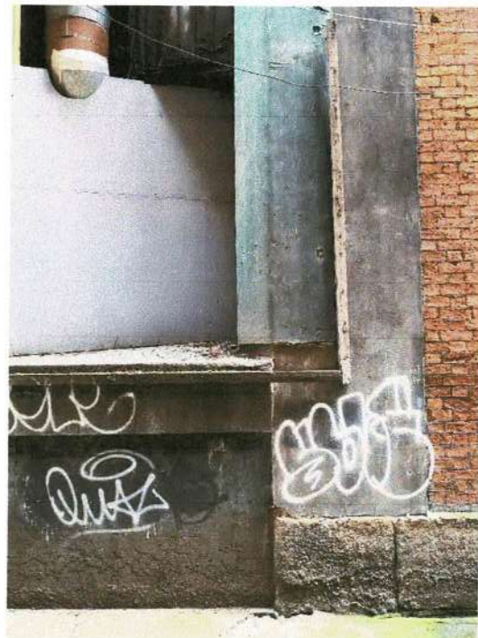
Remove all graffiti. Open up behind boarding when site secured so that extent of repairs can be determined.
