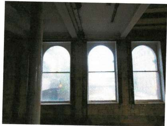
Typical sash windows (previously repaired). Include allowance for easing works.
