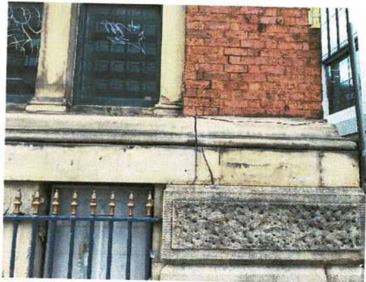
Typical indent repair to stone coursing.
