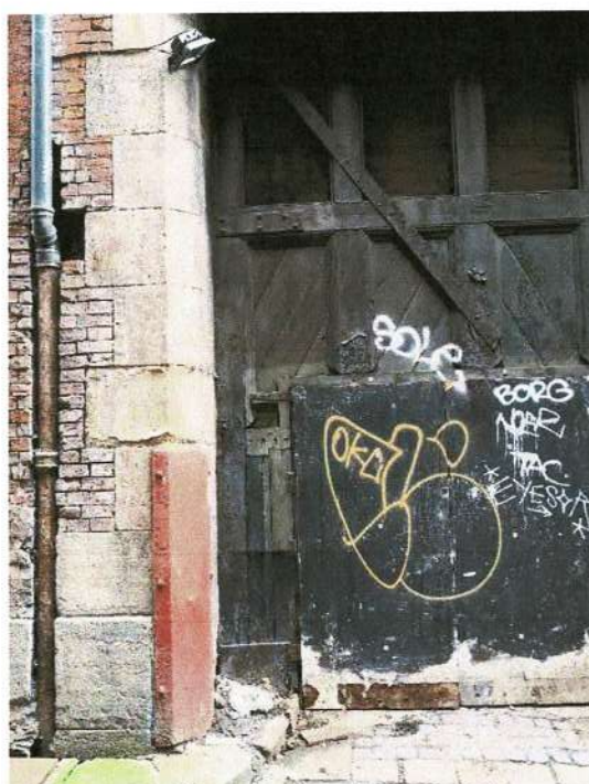
Overhaul loading bay doors and redecorate.
