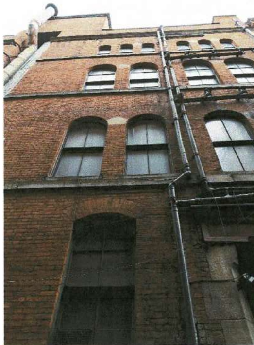
Repoint brickwork to Reyner Street elevation, and replace missing brickwork. See spec and allowance in Schedule of Work
