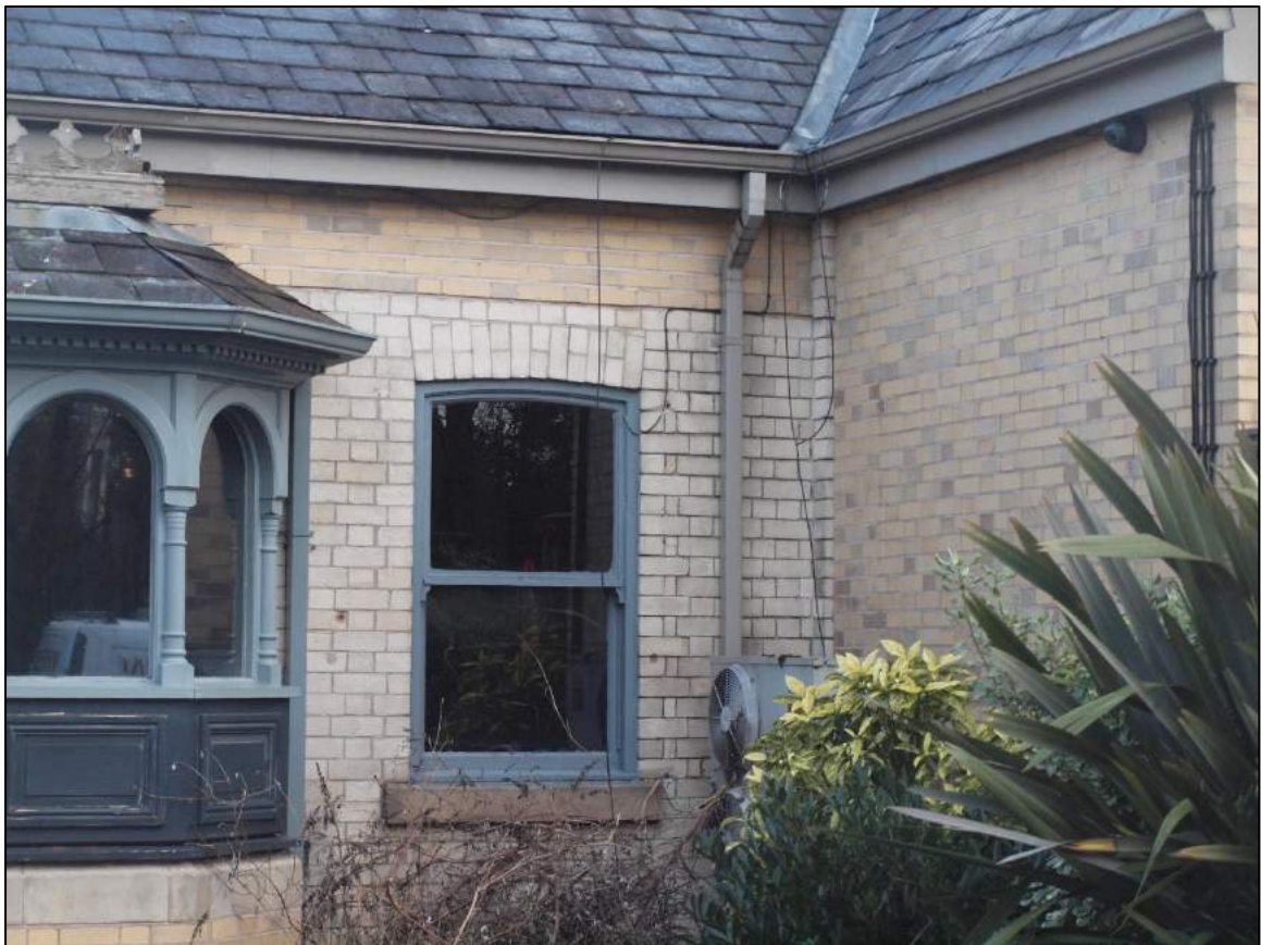
Plate 36: Detail of window and rebuilding
