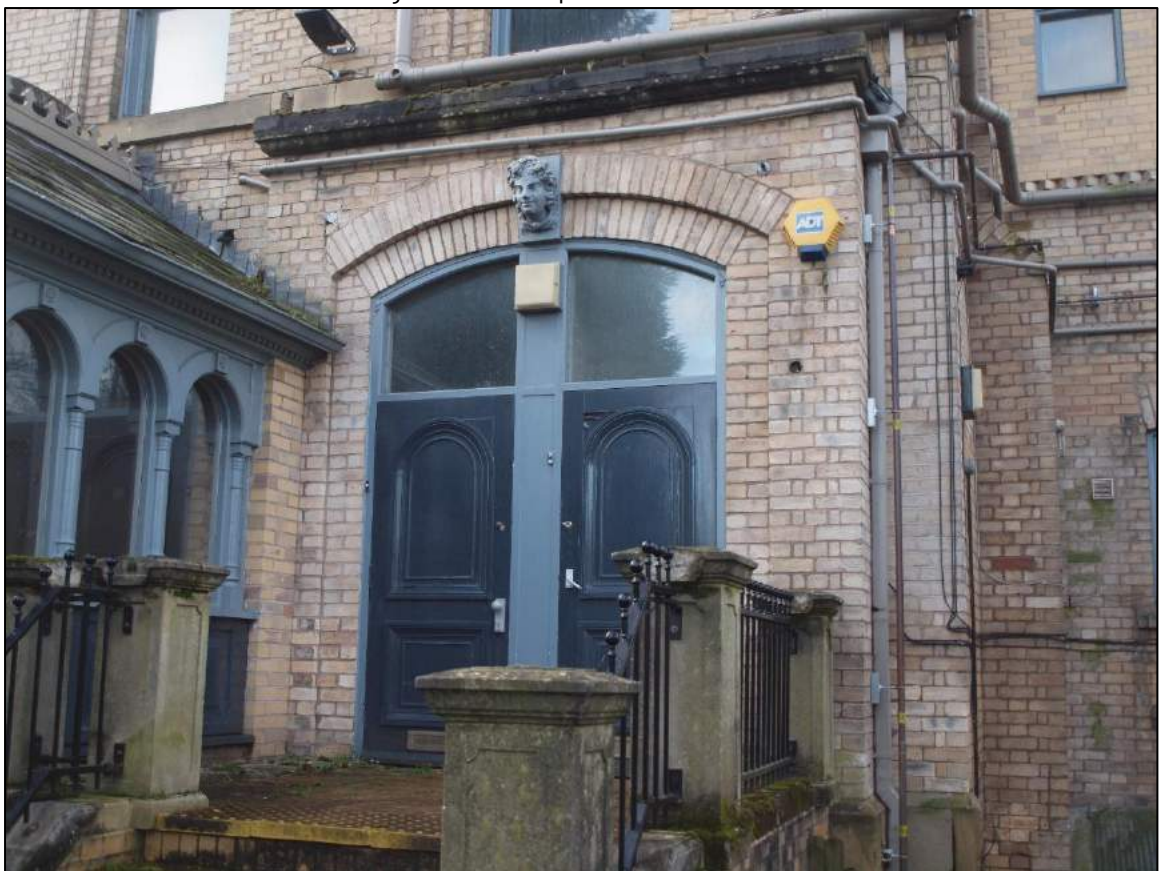
Plate 46: Detail of doorway, formerly a window
