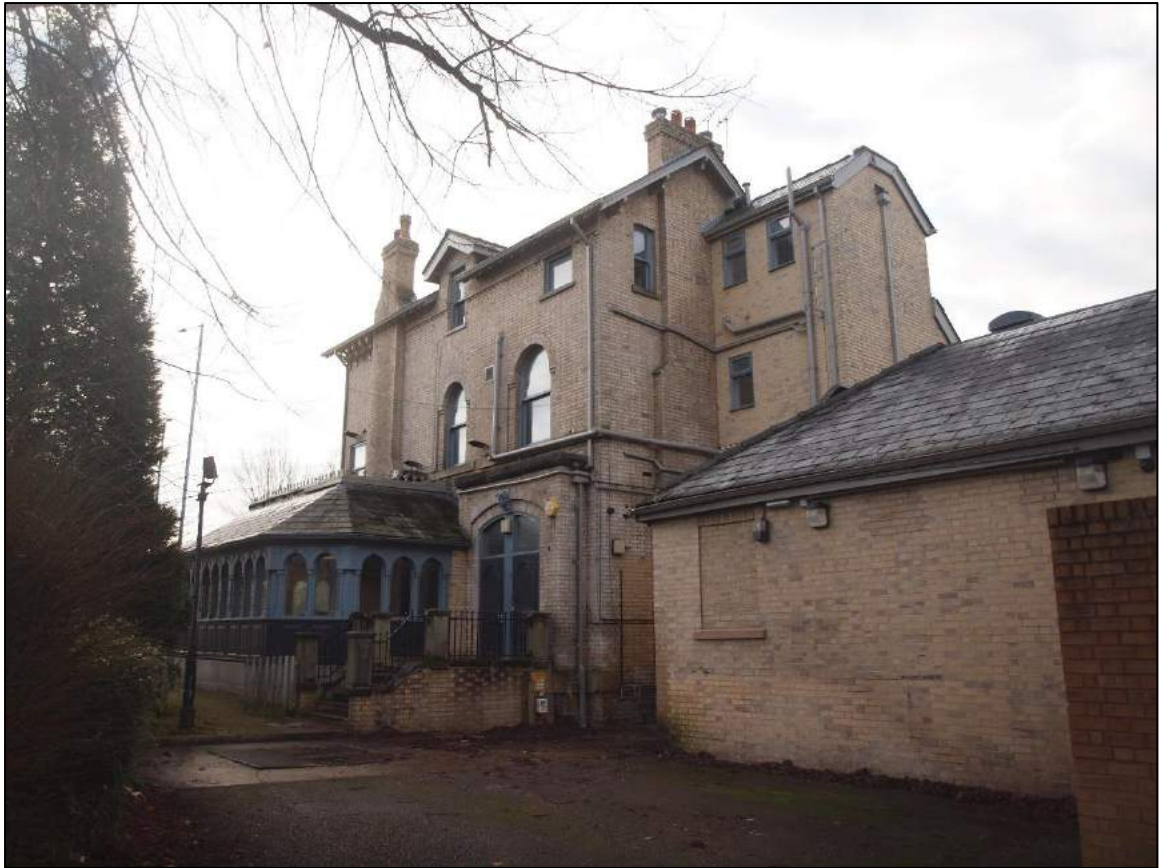
Plate 43: General shot of North east elevation
