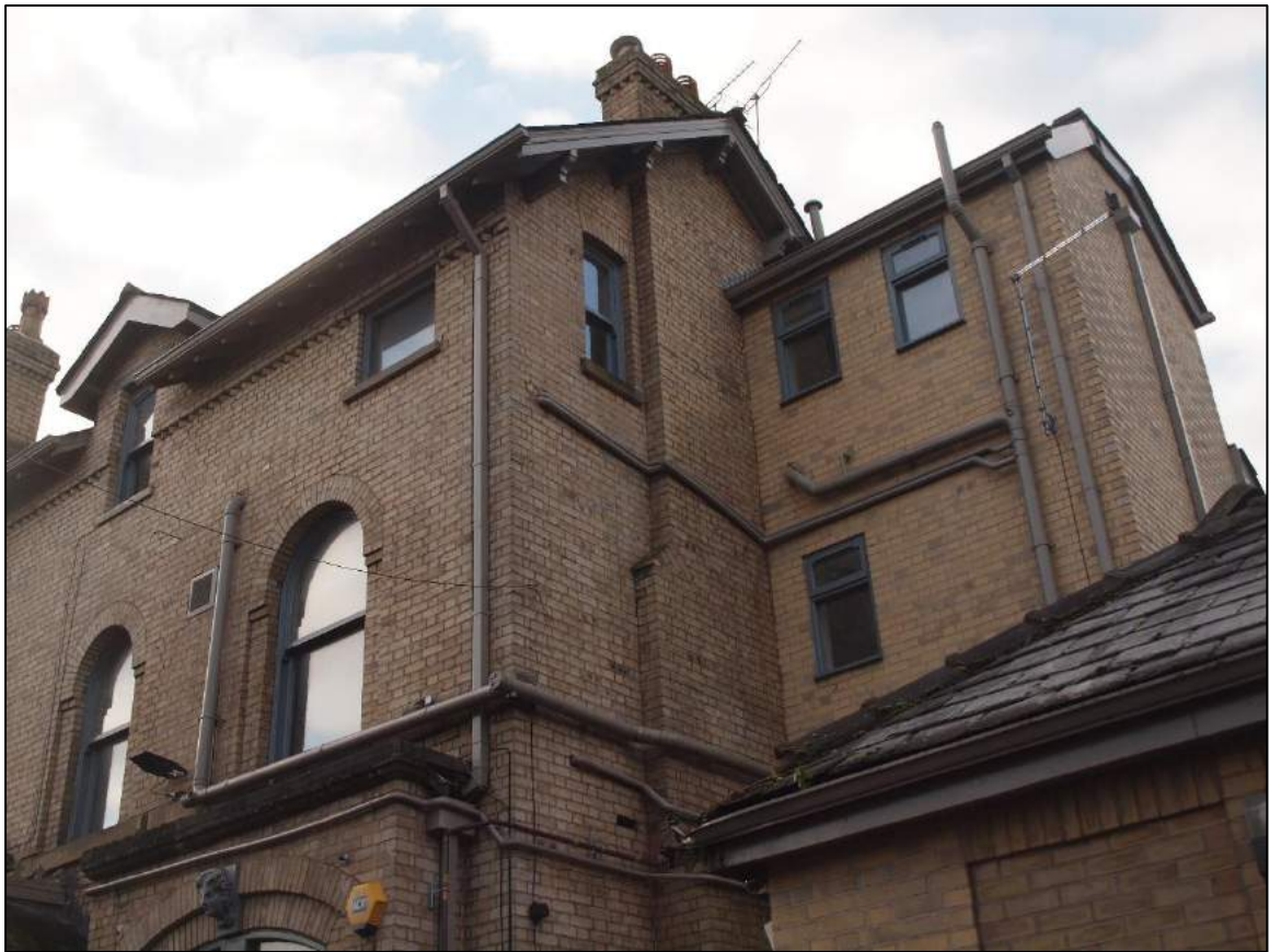
Plate 39: Detail of stair tower
