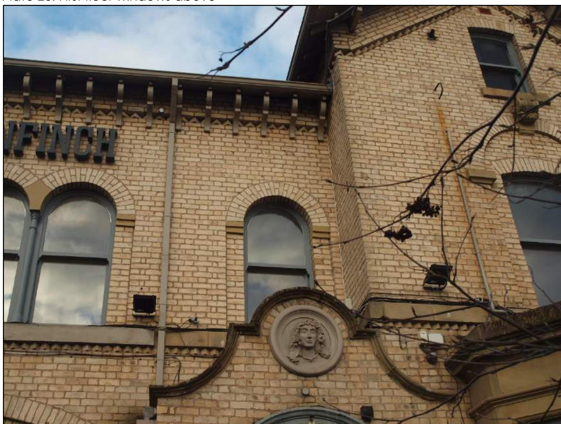
Plate 24: First floor window, central bay
