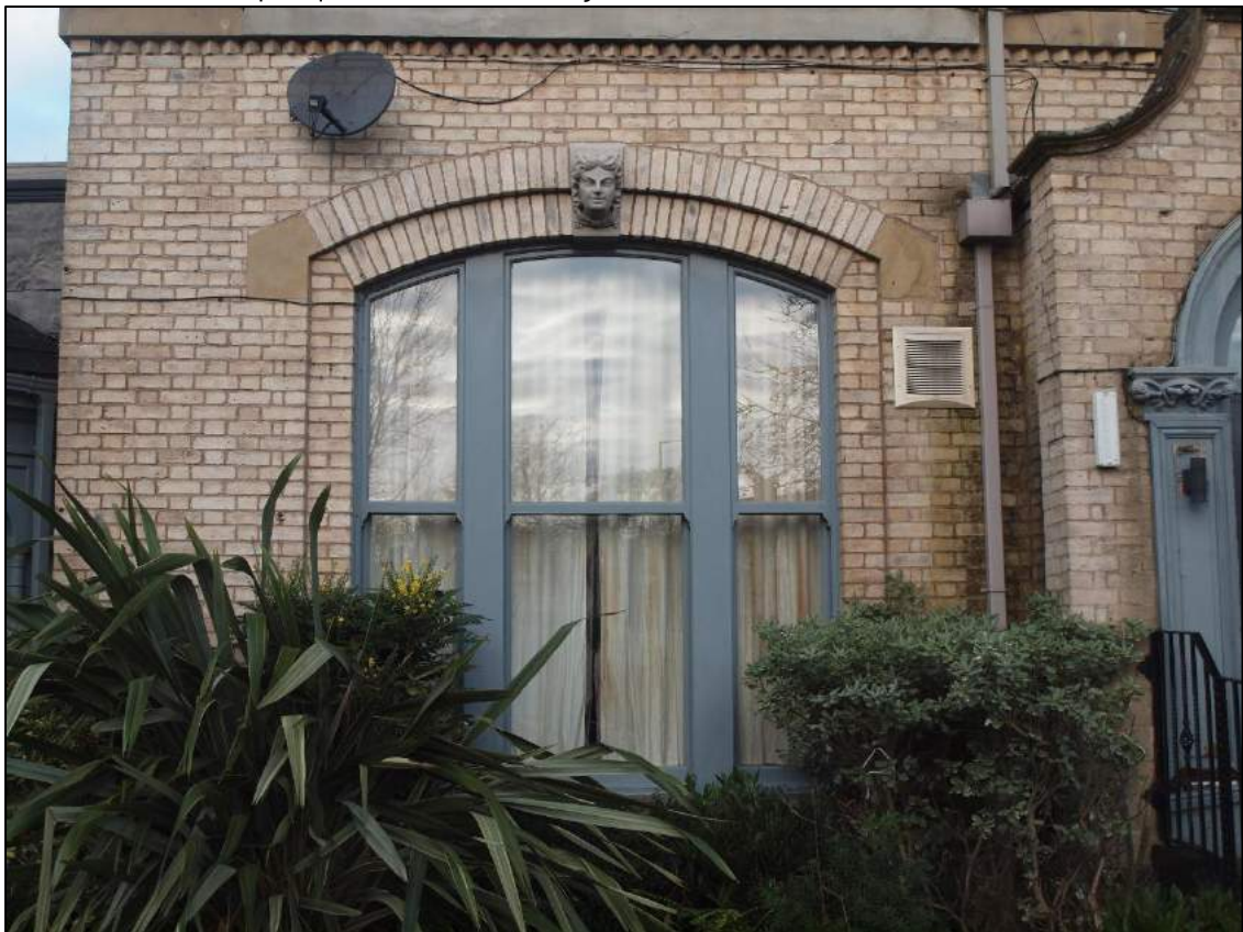
Plate 22: ground floor window in left bay
