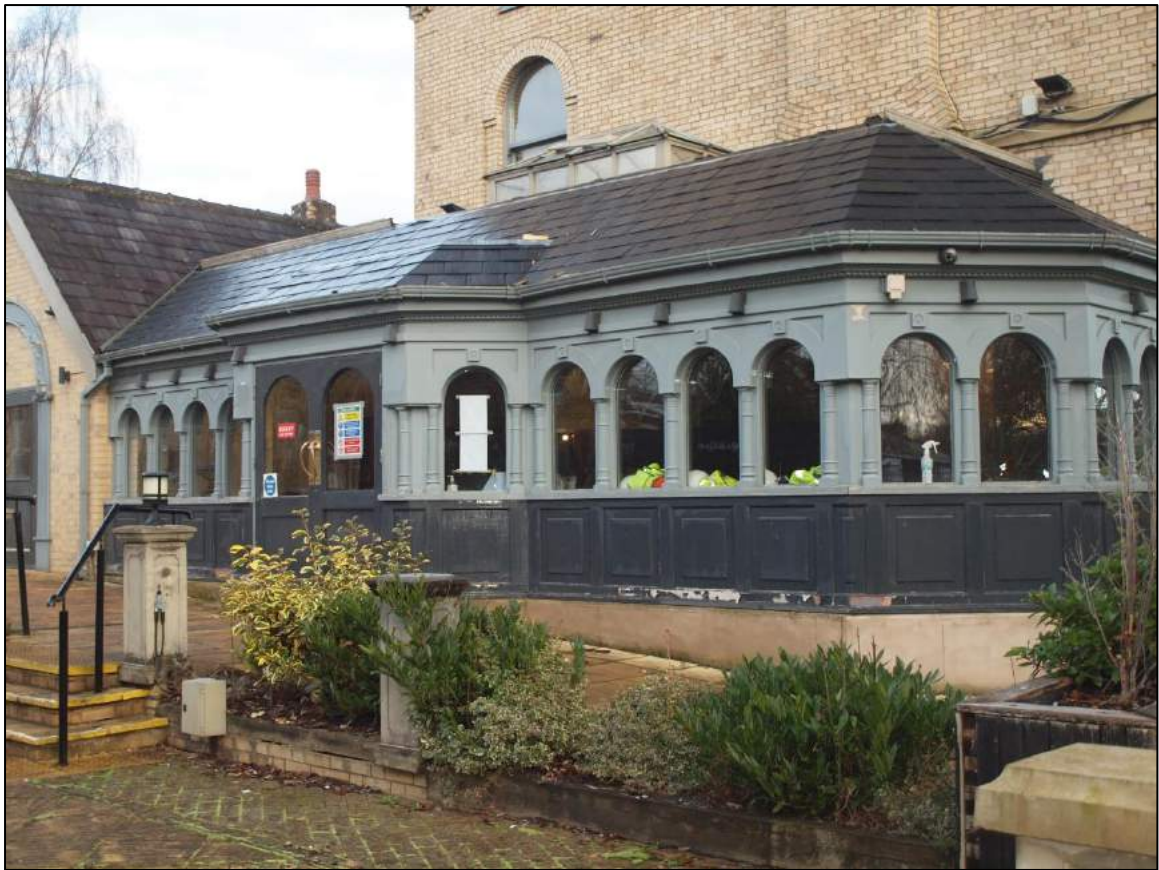
Plate 33: Modern ground floor extension
