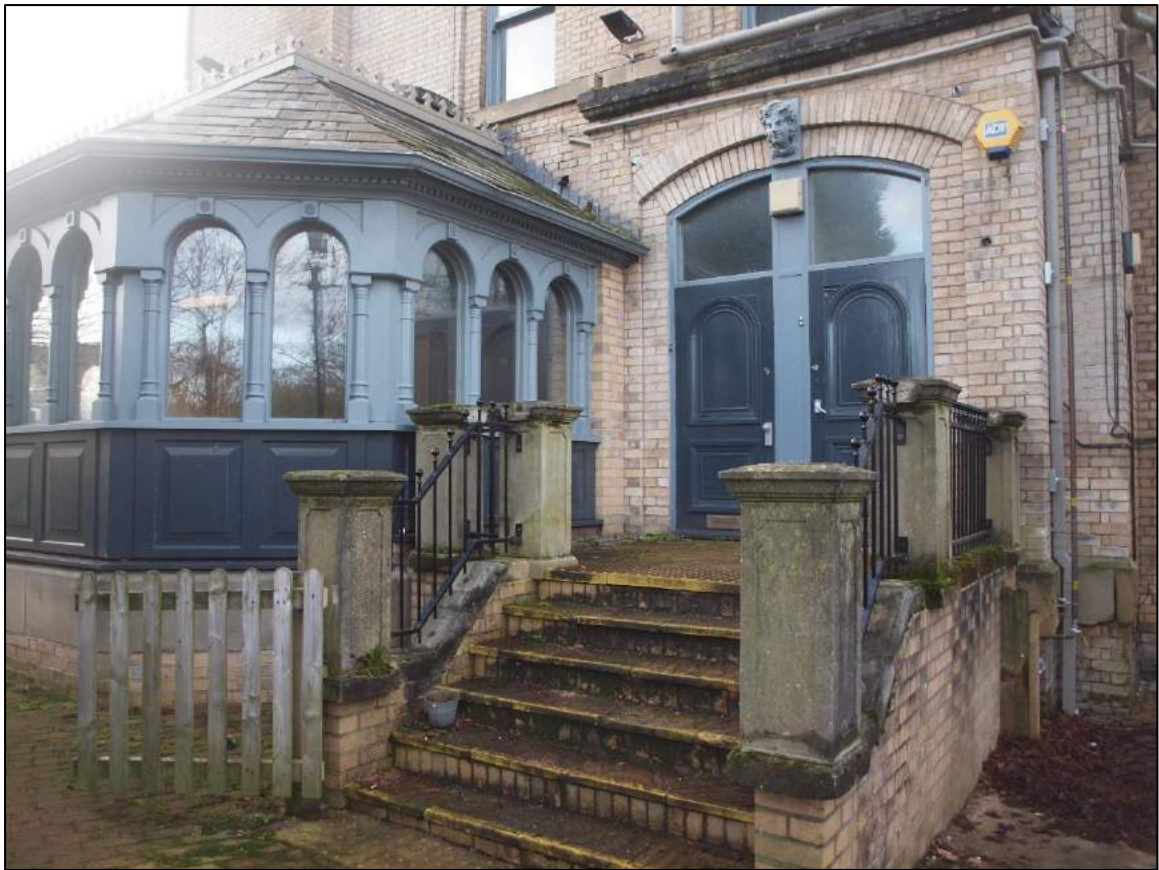
Plate 45: Ground floor doorway with stairs up
