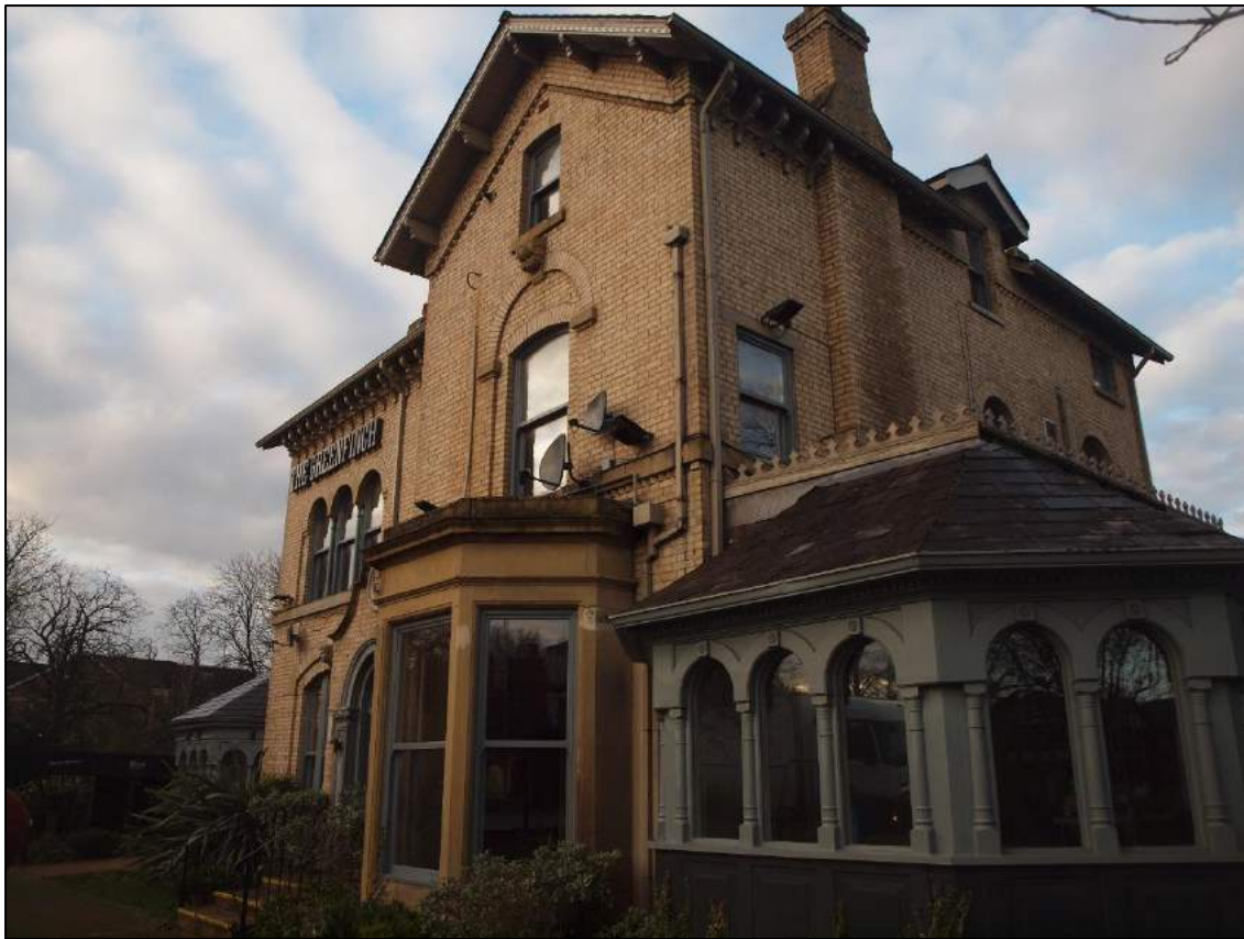
Plate 19: General shot of the southeast elevation
