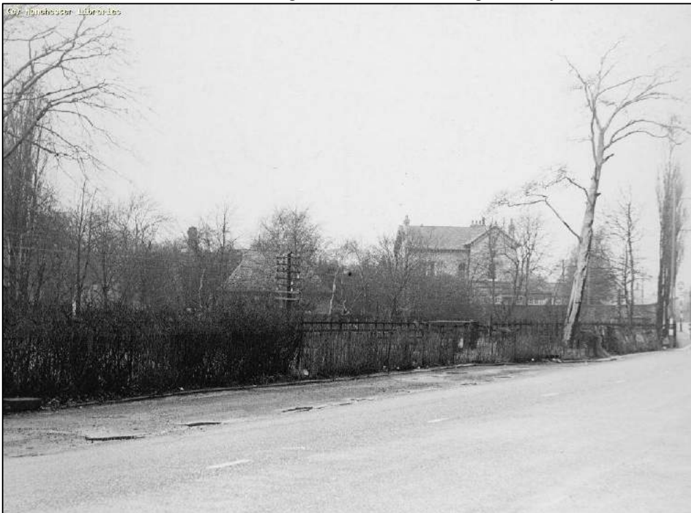
Figure 10: Photograph of the building from 1961 looking north along Palatine Road (Manchester Image Library ref m21920)
