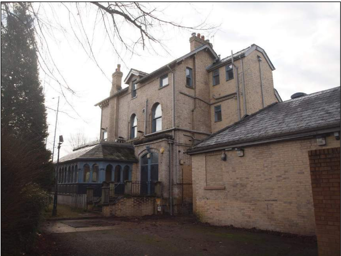
Plate 38: Northwest elevation showing stair tower
