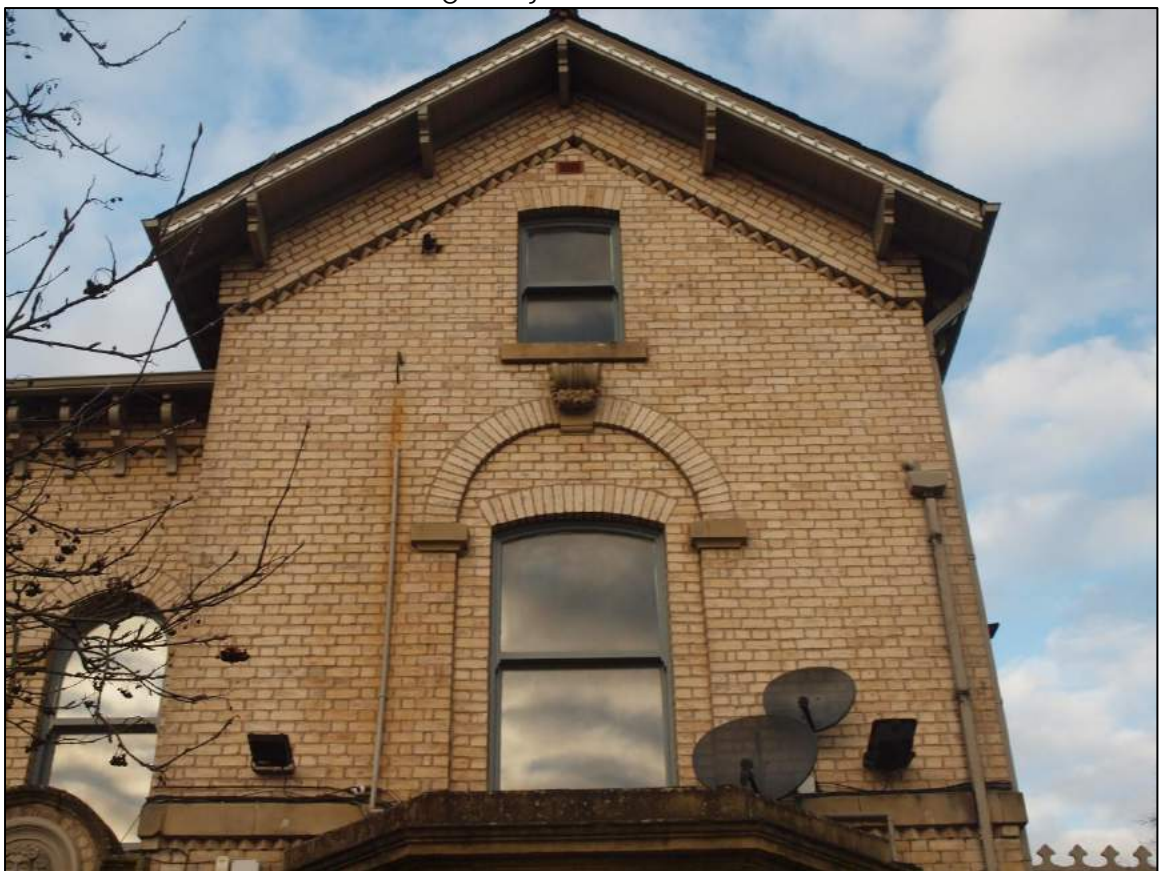
Plate 26: First and attic level window in right bay
