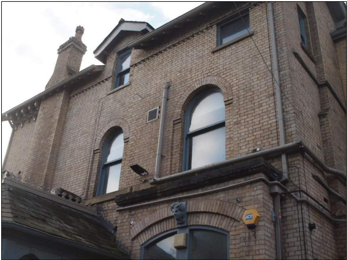
Plate 47: Detail of first and attic floors
