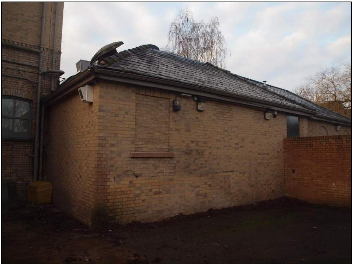
Plate 50: Modern extension to north west
