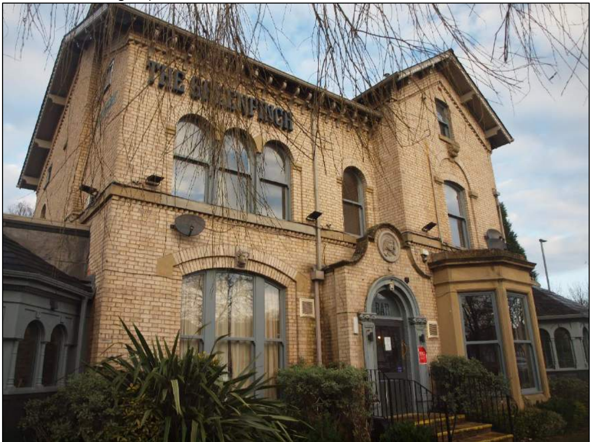
Plate 18: General shot of the southeast elevation
