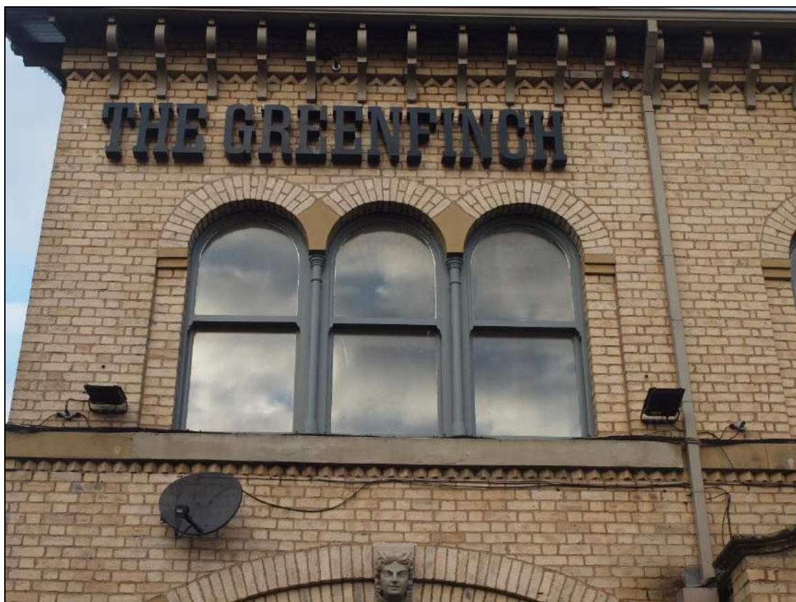
Plate 23: First floor windows above
