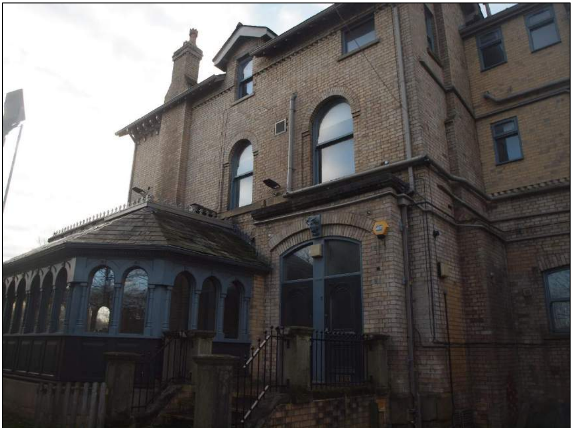
Plate 44: North east elevation of house
