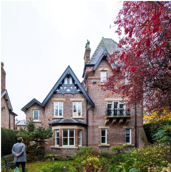
West Elevation of Property
