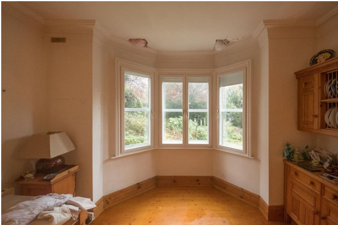
Ground Floor dining room, internal view showing bay window. Locations of intrusive survey investigation visible.
