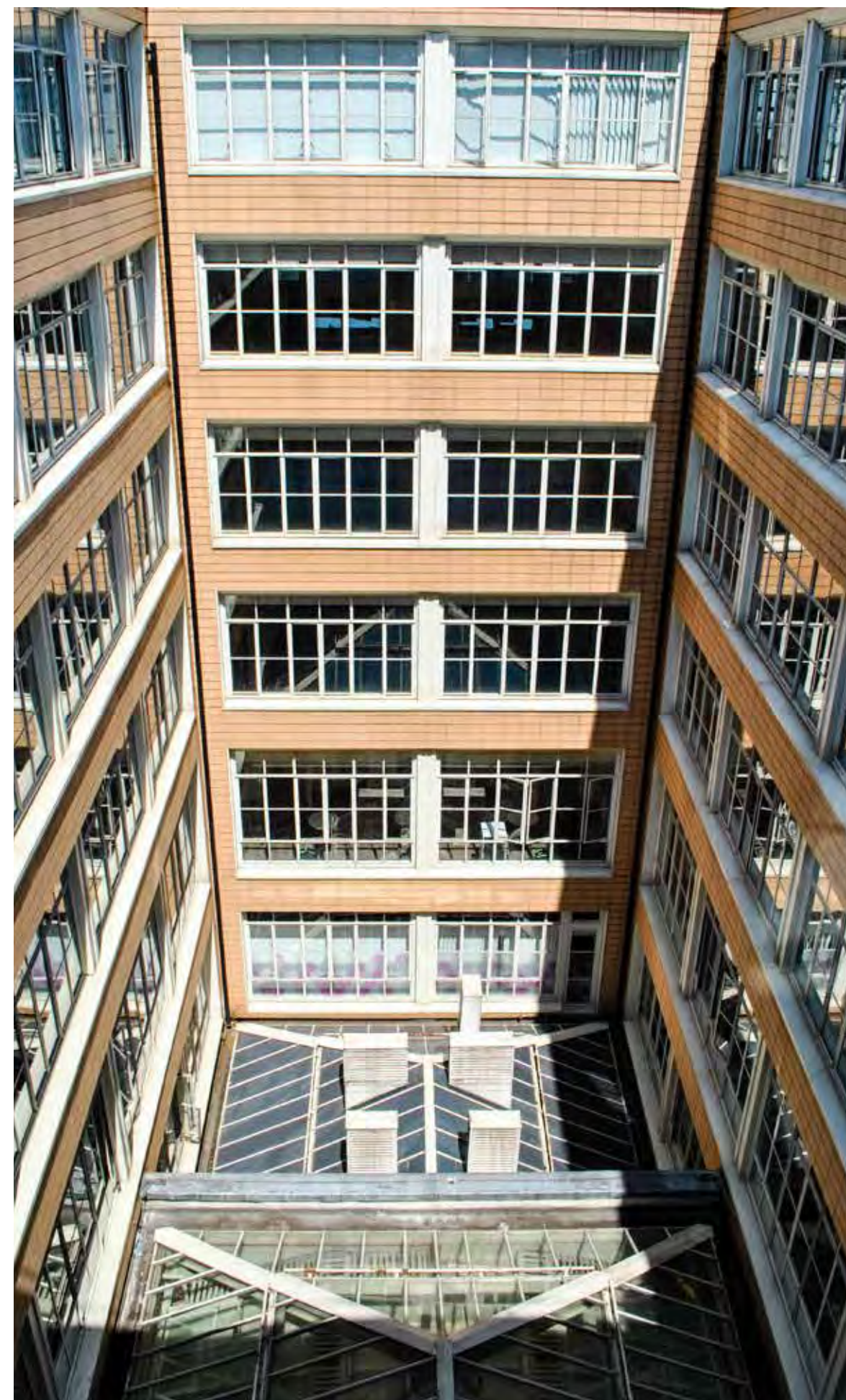
Figure 36 Office Atrium, May 2018.
