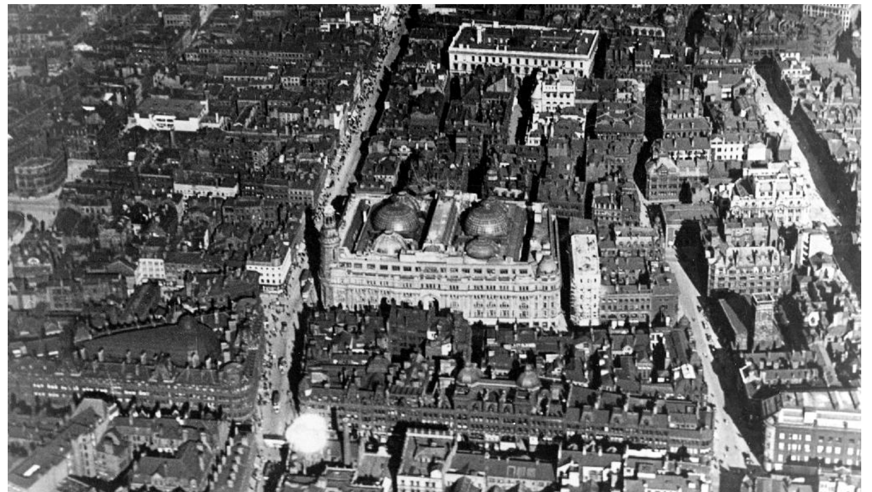
Figure 15 Aerial View of the Royal Exchange (1922) showing 6 domes lighting the whole of the trading hall. © Manchester Libraries
