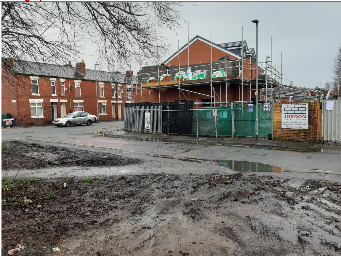
Photograph 4: Access noted within the north-east of the site
