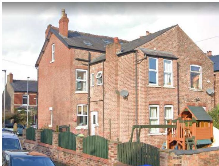
Rear elevation showing unique bay windows to outrigger
