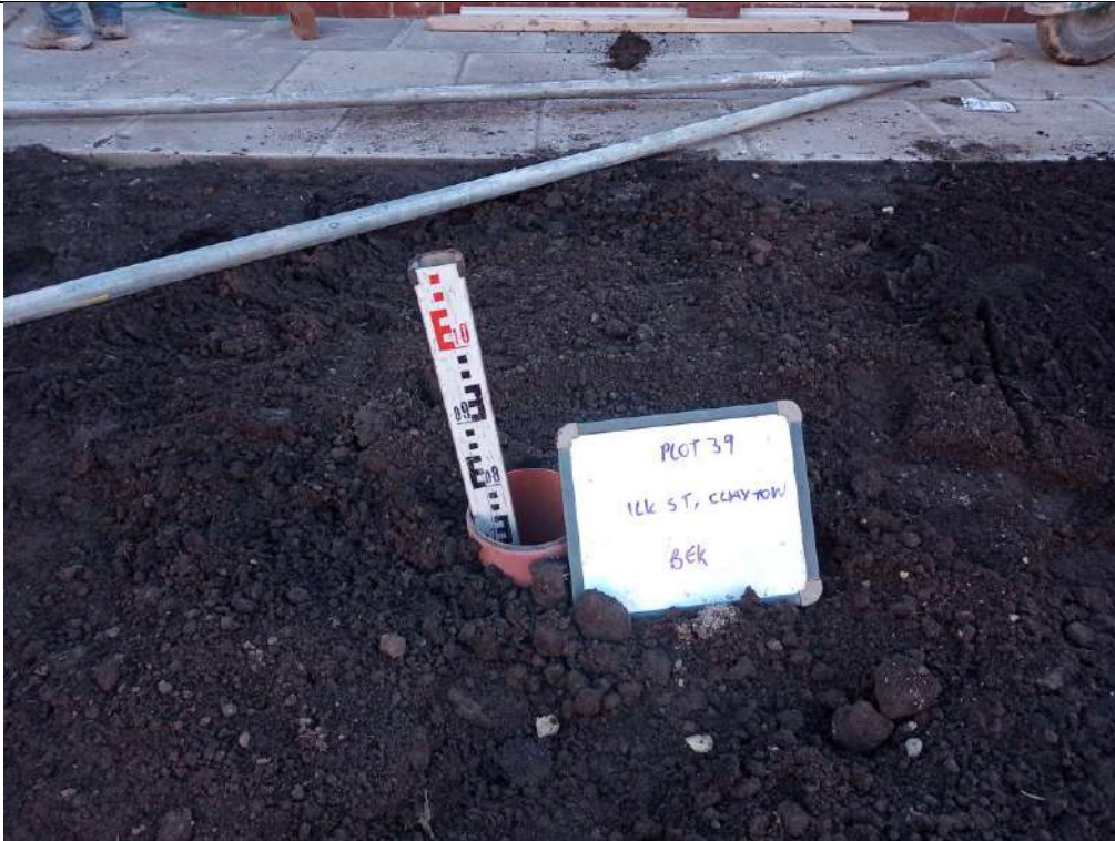
Photograph 1: Validation of Garden Capping Thickness
