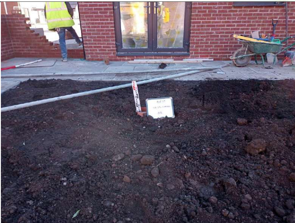
Photograph 2: Validation of Garden Capping Thickness
