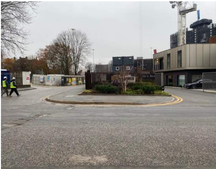
11. Melbourne St, off Great Jackson St. Currently used as main access road to Renaker's Crown St project..
