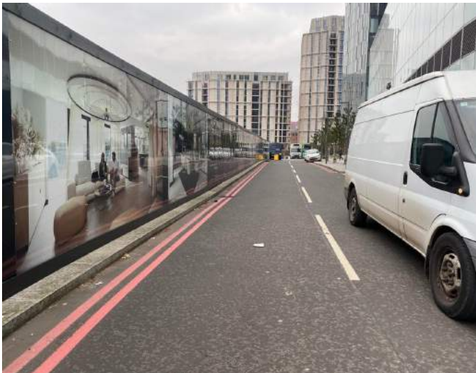
23. Owen St, along eastern boundary of Plot E. Kerbs installed as part of Deansgate Square development.
