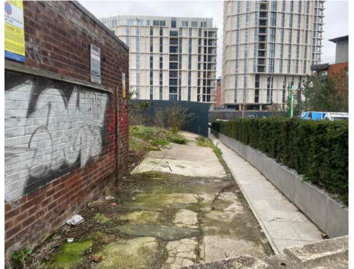
26. Interface between Owen St and site boundary of Plot B.
