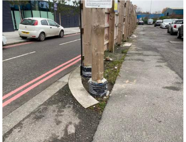
30. Existing hardworks behind Transition hoarding inside site boundaries.
