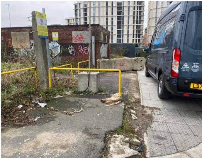
27. Paving outside entrance to Plot E along Owen St.
