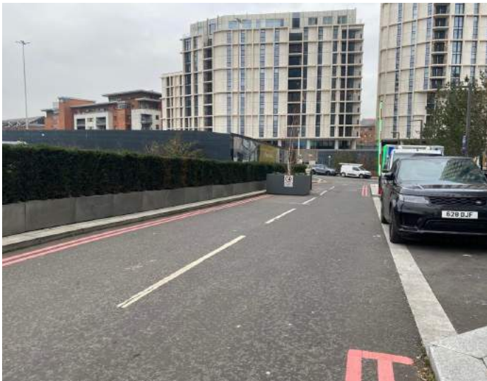
31. New paving and kerbing along Owen St.
