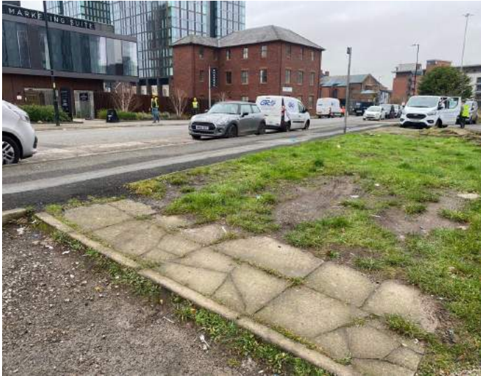
13. Existing hardworks to western site boundary along Great Jackson St.
