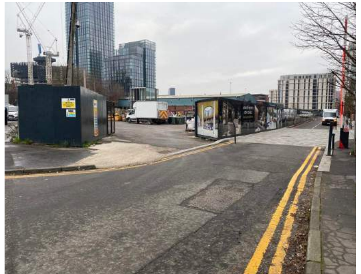
20. Access to Owen St from Great Jackson St. Showing entrance access to Plot F, to south of Plot E site boundary.
