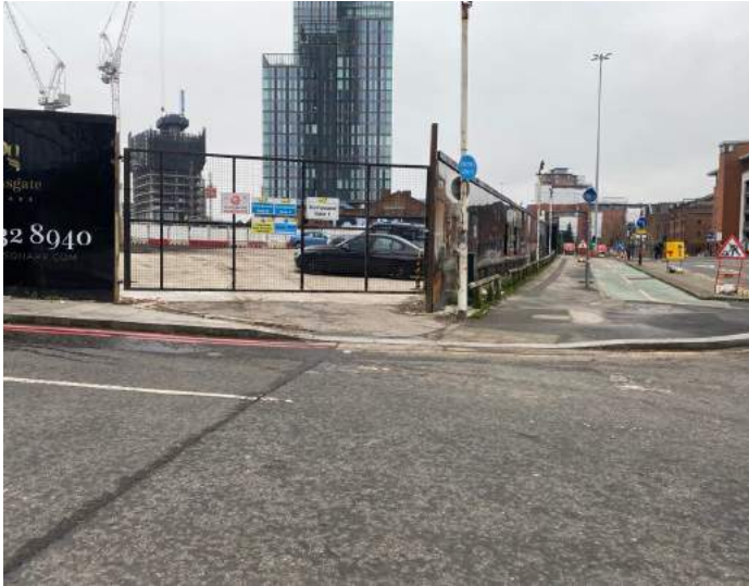
33. Access gate to Plot B at junction of Owen St, Deansgate and Chester Rd.
