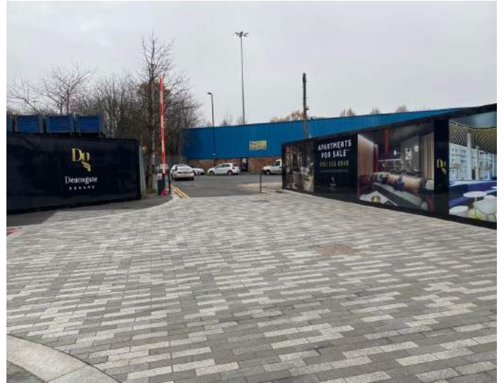
22. View from Owen St showing restricted access and new paving finishes from Deansgate Square development.
