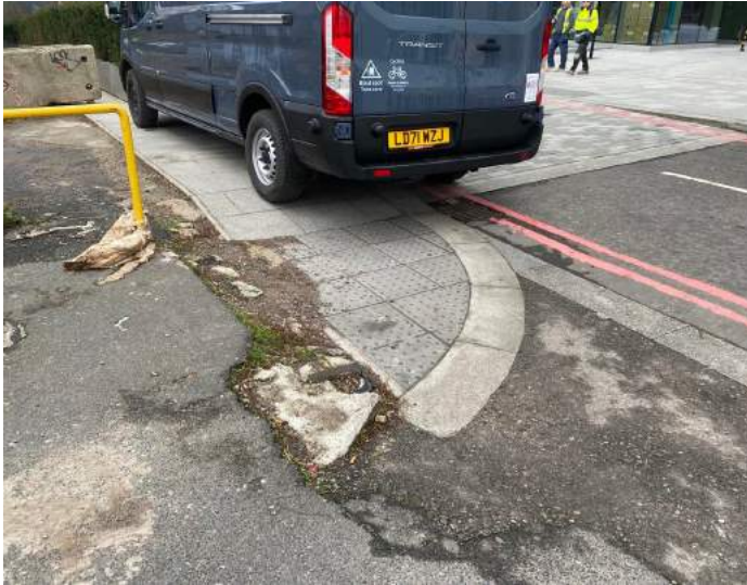
29. Interface between Plot E site boundary and new paving from Deansgate Square development.
