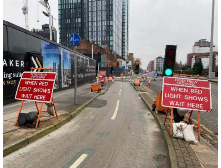
38. Existing roadworks to Plot B northern site boundary at junction of Chester Rd and Great Jackson St.
