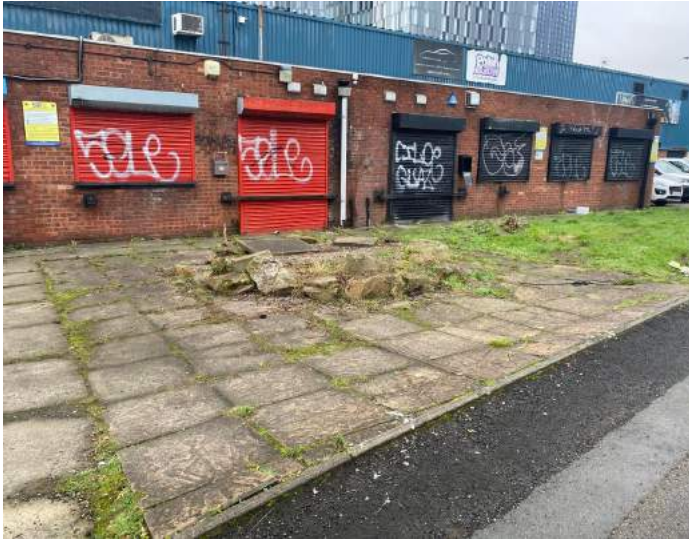
9. Existing building on Transition Plot E site.
