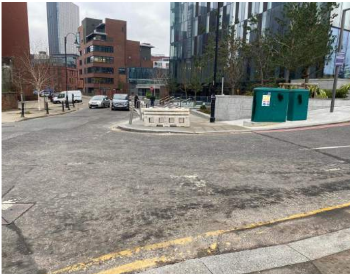
35. Existing highway at junction of Owen St and Deansgate.
