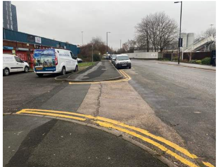
6. Access point to Transition site from Great Jackson St.
