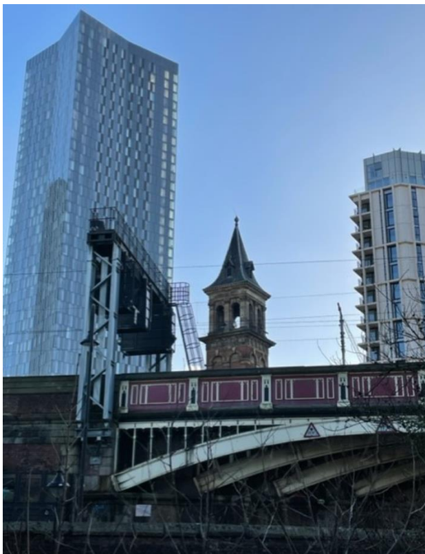
Fig 64. View 4 Rochdale Canal
