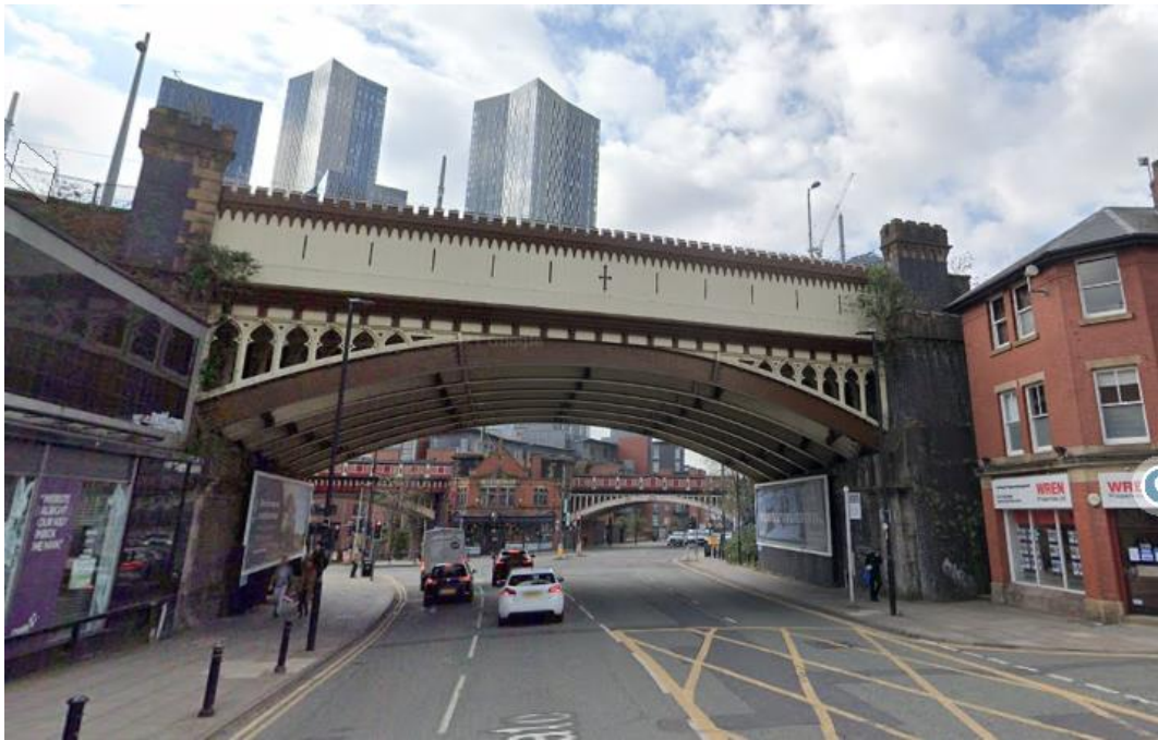
Fig 13 Castlefield Railway Viaduct
