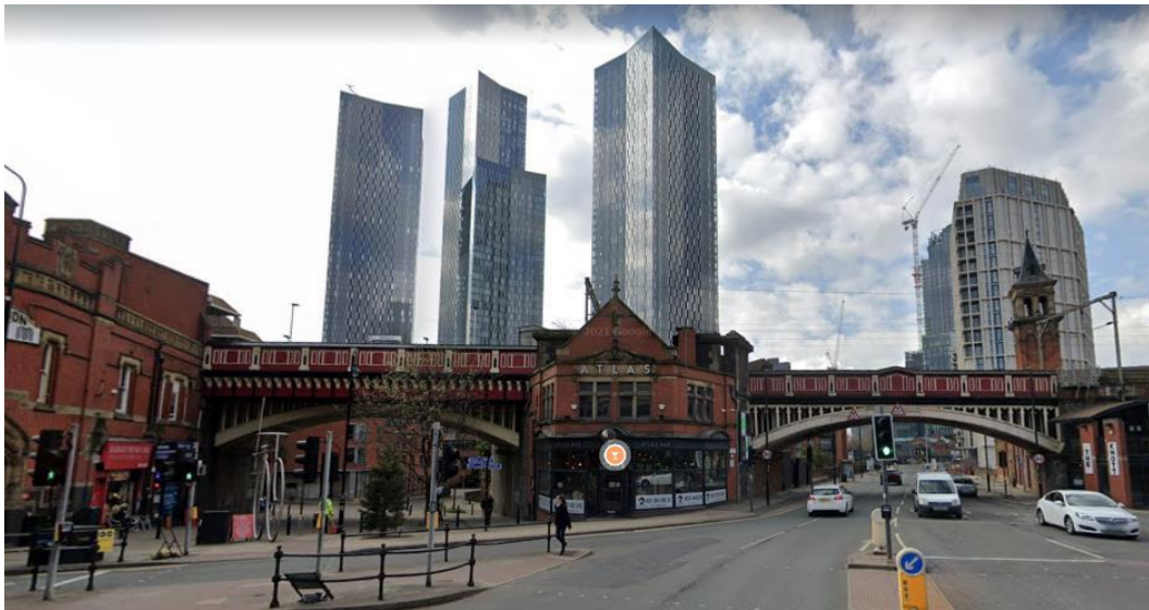
Fig 28. View 2 Deansgate looking from East to West in front of MSJ and AR Viaduct.
