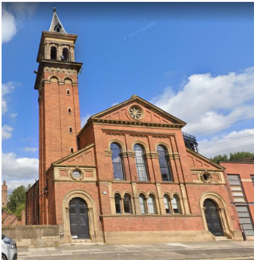
Fig 11. Former Congregational Chapel
