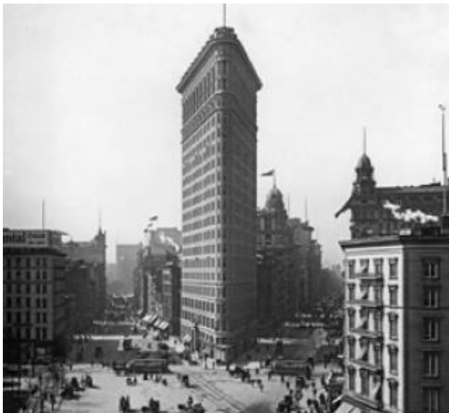
Fig 49. Flat Iron building in New York
