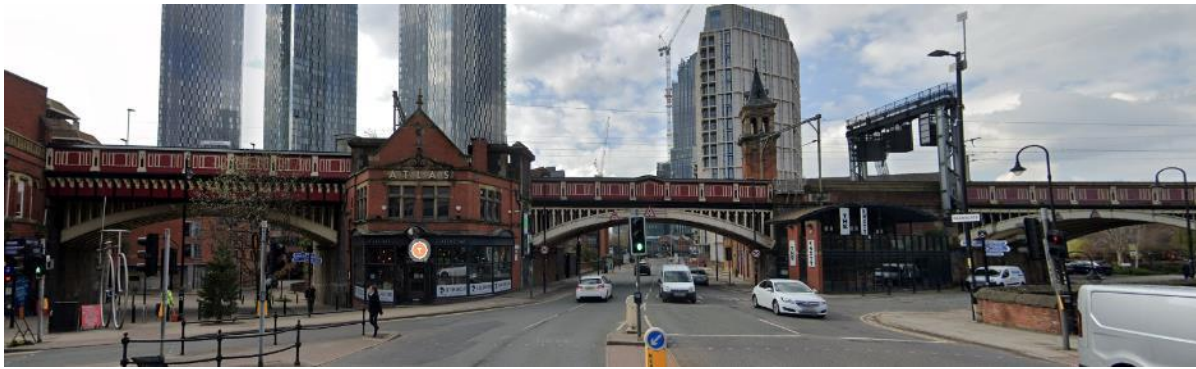
Fig 14. Manchester South Junction and Altrincham Railway Viaduct (MSJ & AR).
