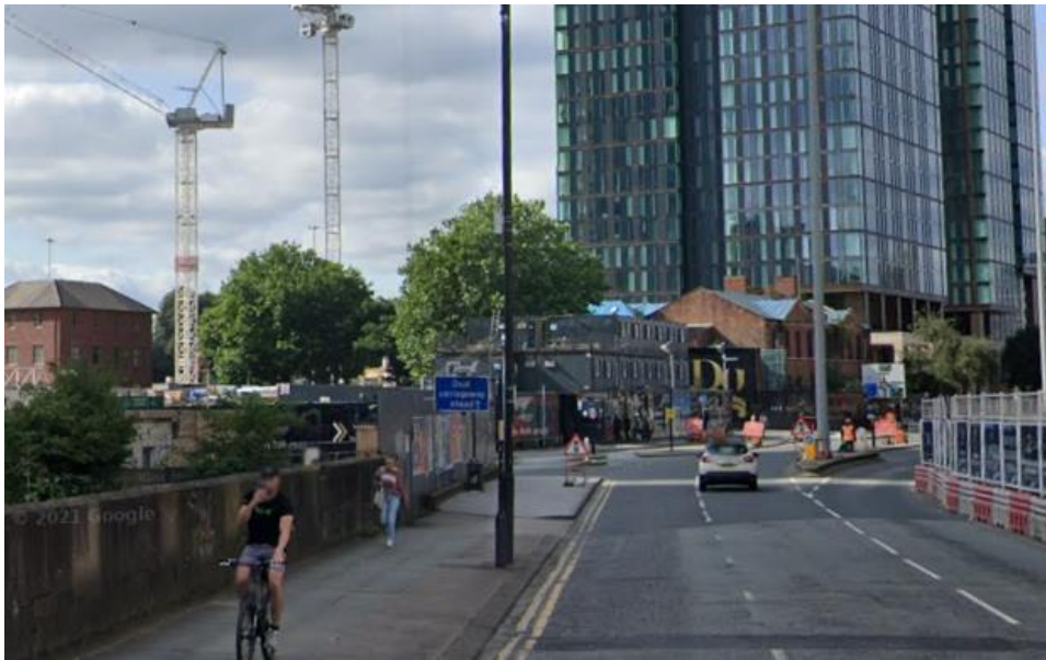
Fig 58. View from Bridgewater Viaduct looking east
