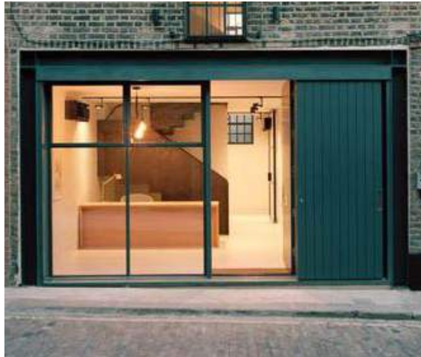
Retail shopfront recessed from brick facade
