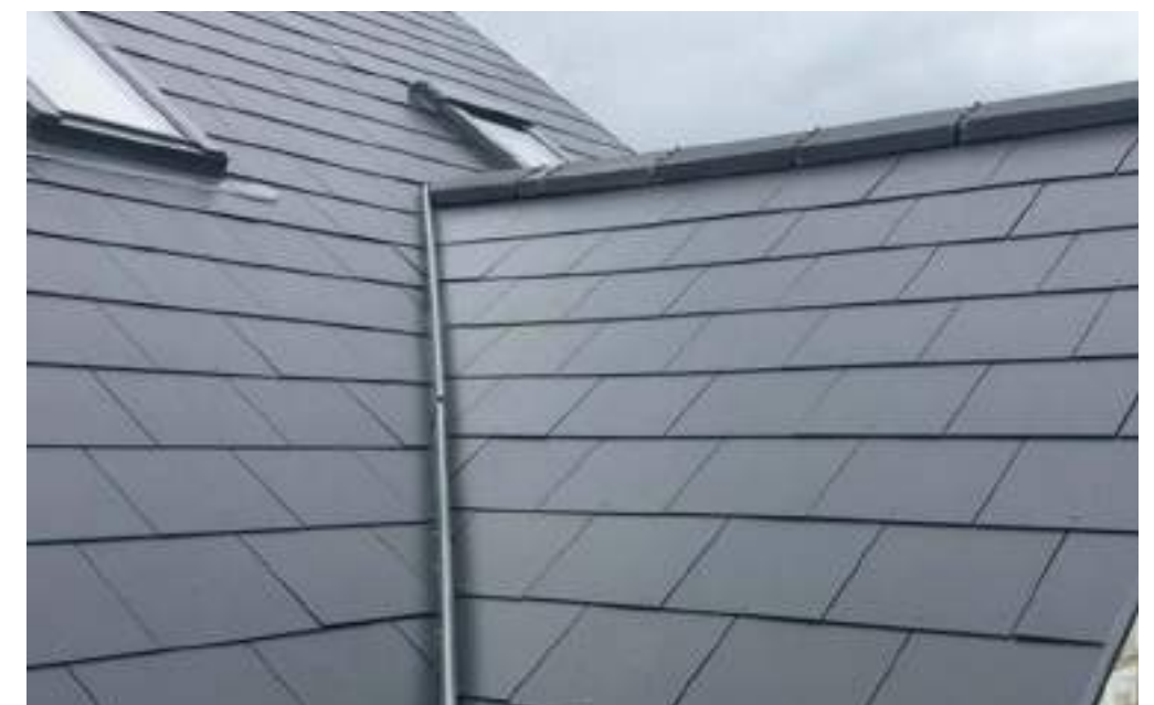
Fibre Cement Roof Tiles to houses
