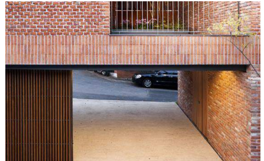
Feature brick detail above shopfronts
