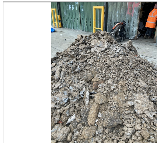
Trial Pit 311 Spoil
