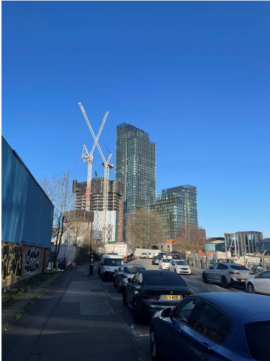
Figure 7-1 - Crown Street Development Under Construction (14th March 2022)
