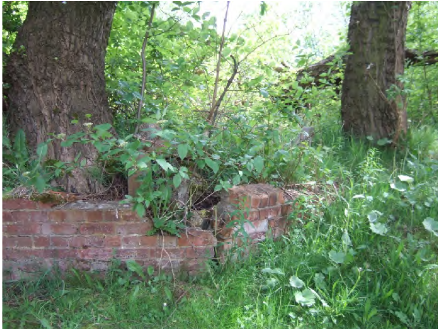
Photograph 7: Adjacent to the Rochdale Canal (south-west facing)
