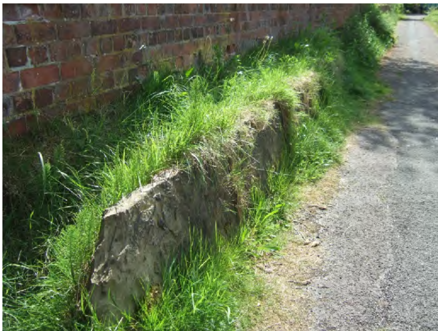
Photograph 6: Adjacent to the Rochdale Canal (west facing)
