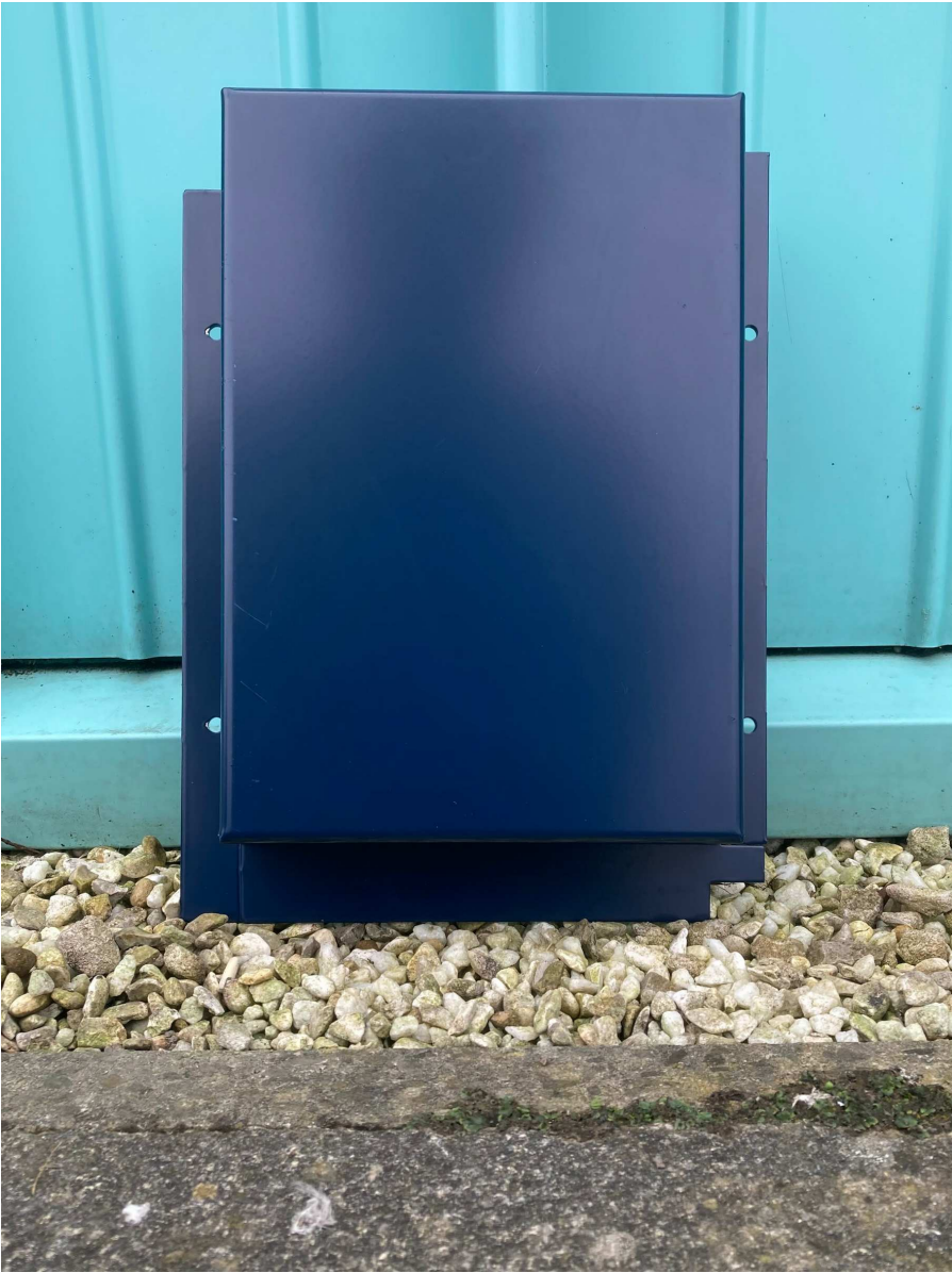
External canopy cladding. RFL brand colour. PANTONE 289 / RAL 5026
