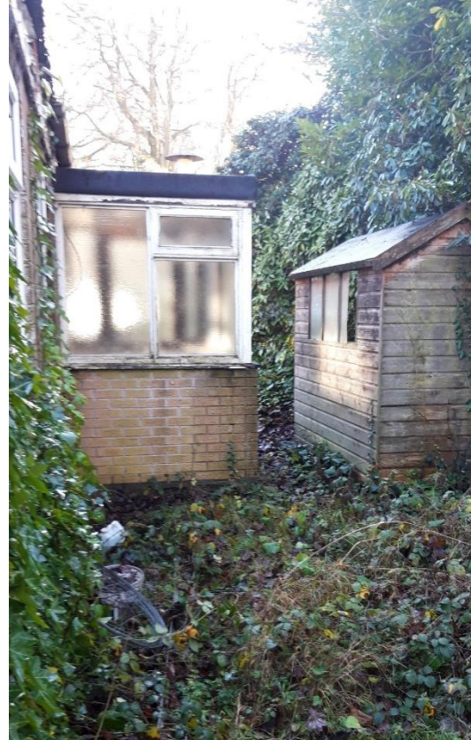
Rear of the house:
