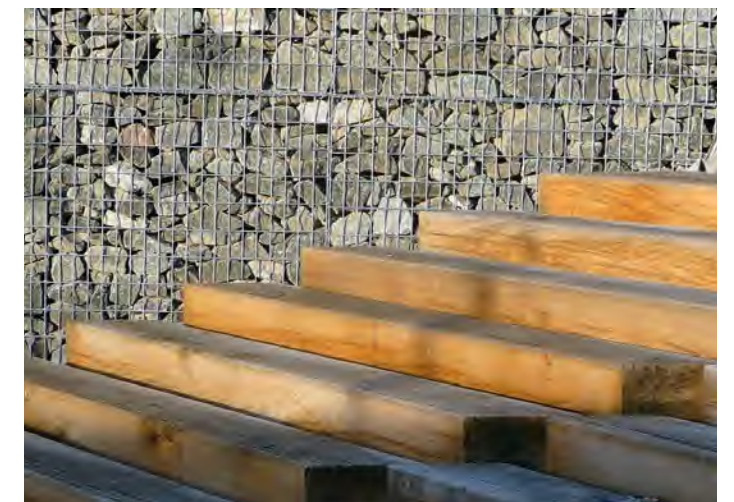
GABIONS AND TIMBER DETAILING TO RED BANK TERRACES
