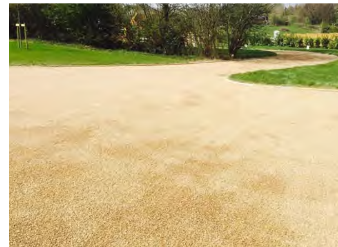
RESIN BONDED GRAVEL TO ST CATHERINE'S WOOD PATHS
