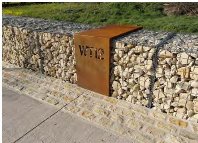
GABIONS RETAINING ELEMENTS WITH BESPOKE DETAILING
