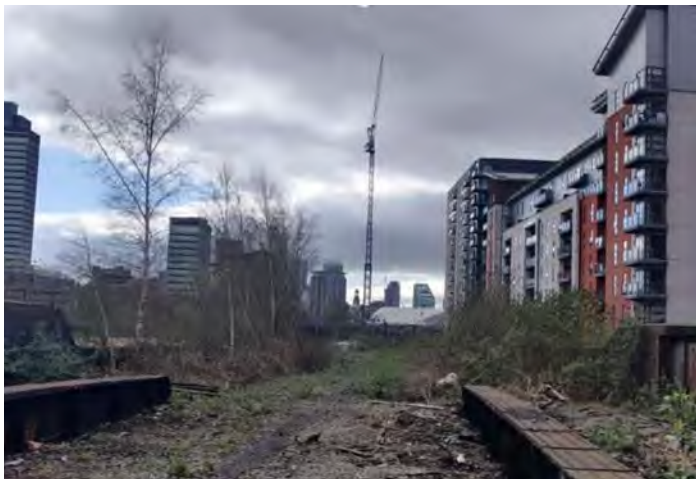
VIEW LOOKING TOWARDS THE CITY CENTRE ALONG THE OLD VIADUCT - GROUP G11 - INACCESSIBLE SMALL TREES ON OLD VIADUCT.
