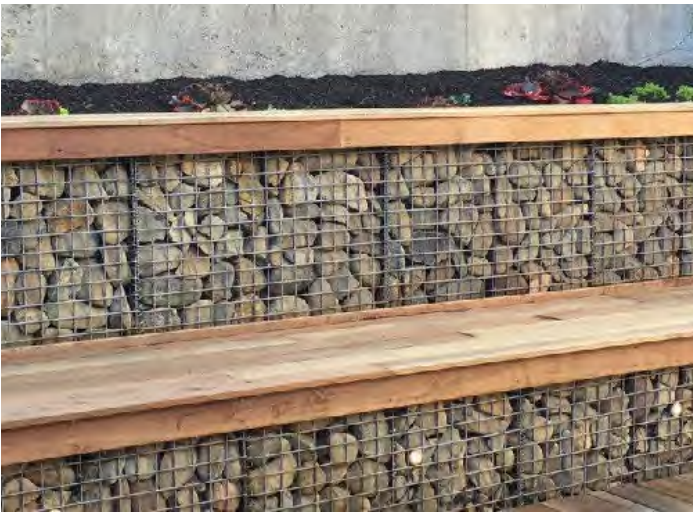
TIMBER TOPPED GABION SEATS TO RED BANK TERRACES
