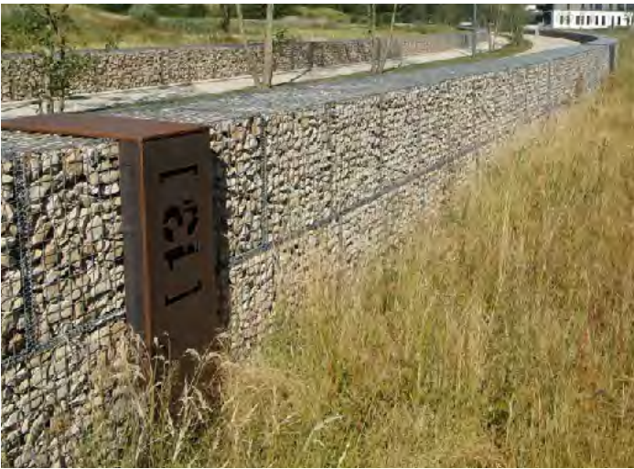
GABION RETAINING WALLS WITH BESPOKE DETAILING
