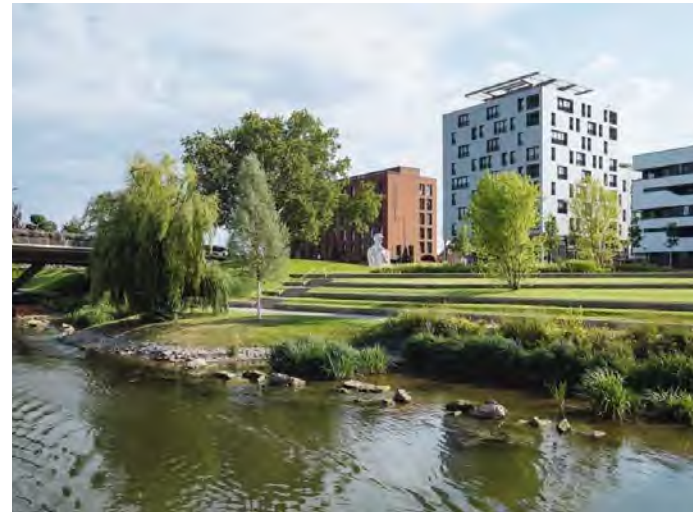
RIP RAP BOULDERS AND PLANTING TO NEW RIVER BANKS
