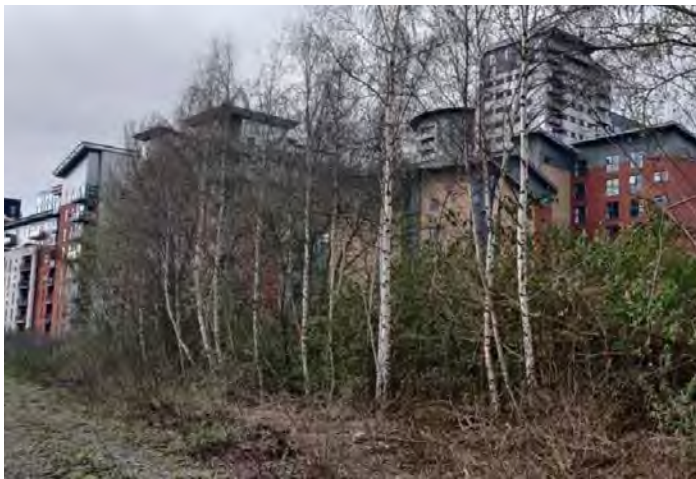
VIEW NORTH LOOKING AT GROUP G10 - BOUNDARY TREES GROWING ON THE OLD VIADUCT
