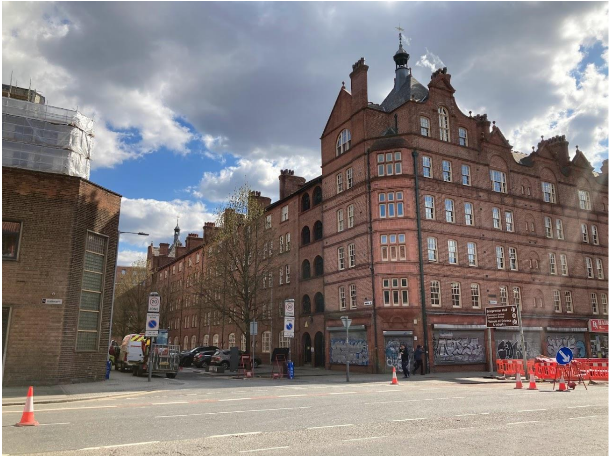
FIGURE 16 – OLDHAM ROAD EXTERNAL ELEVATION
