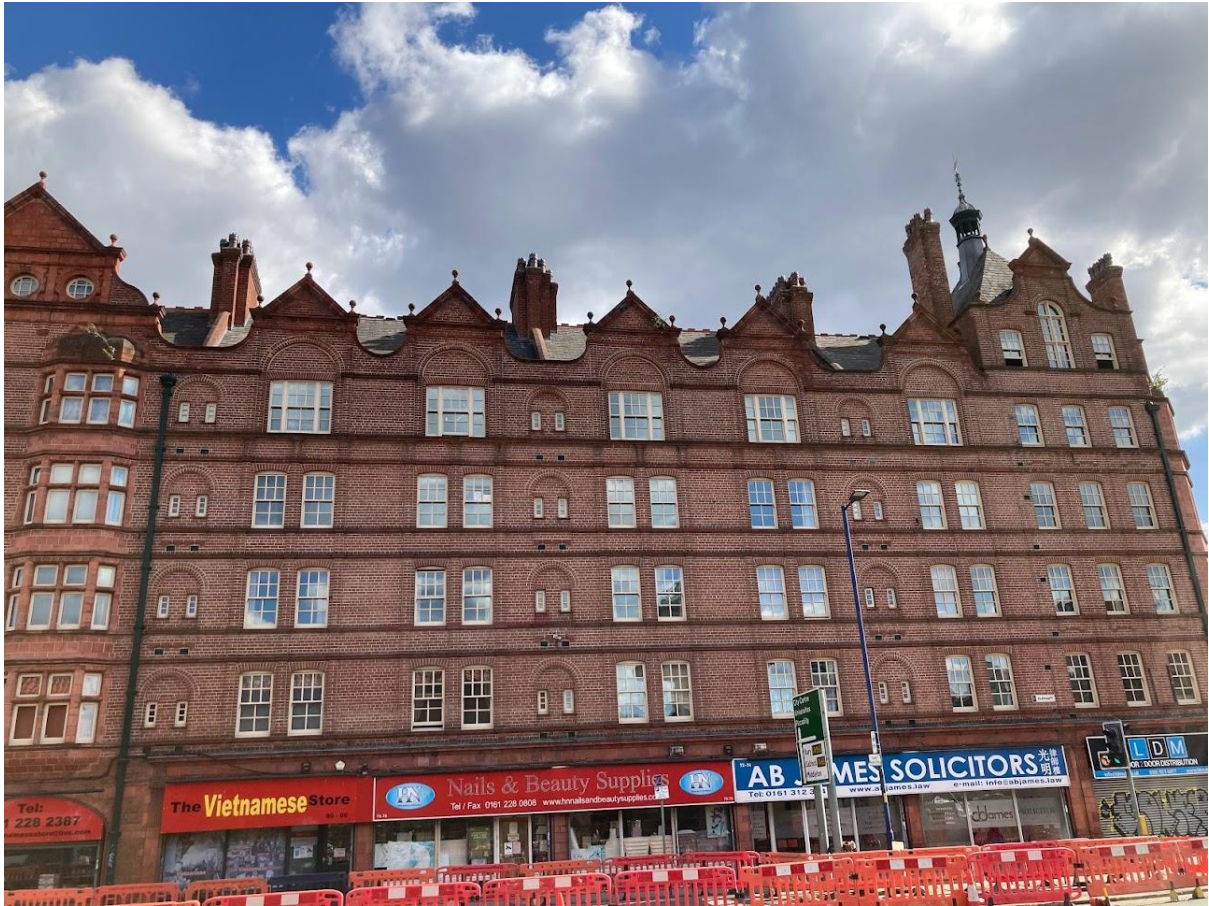
FIGURE 14 – OLDHAM ROAD EXTERNAL ELEVATION
