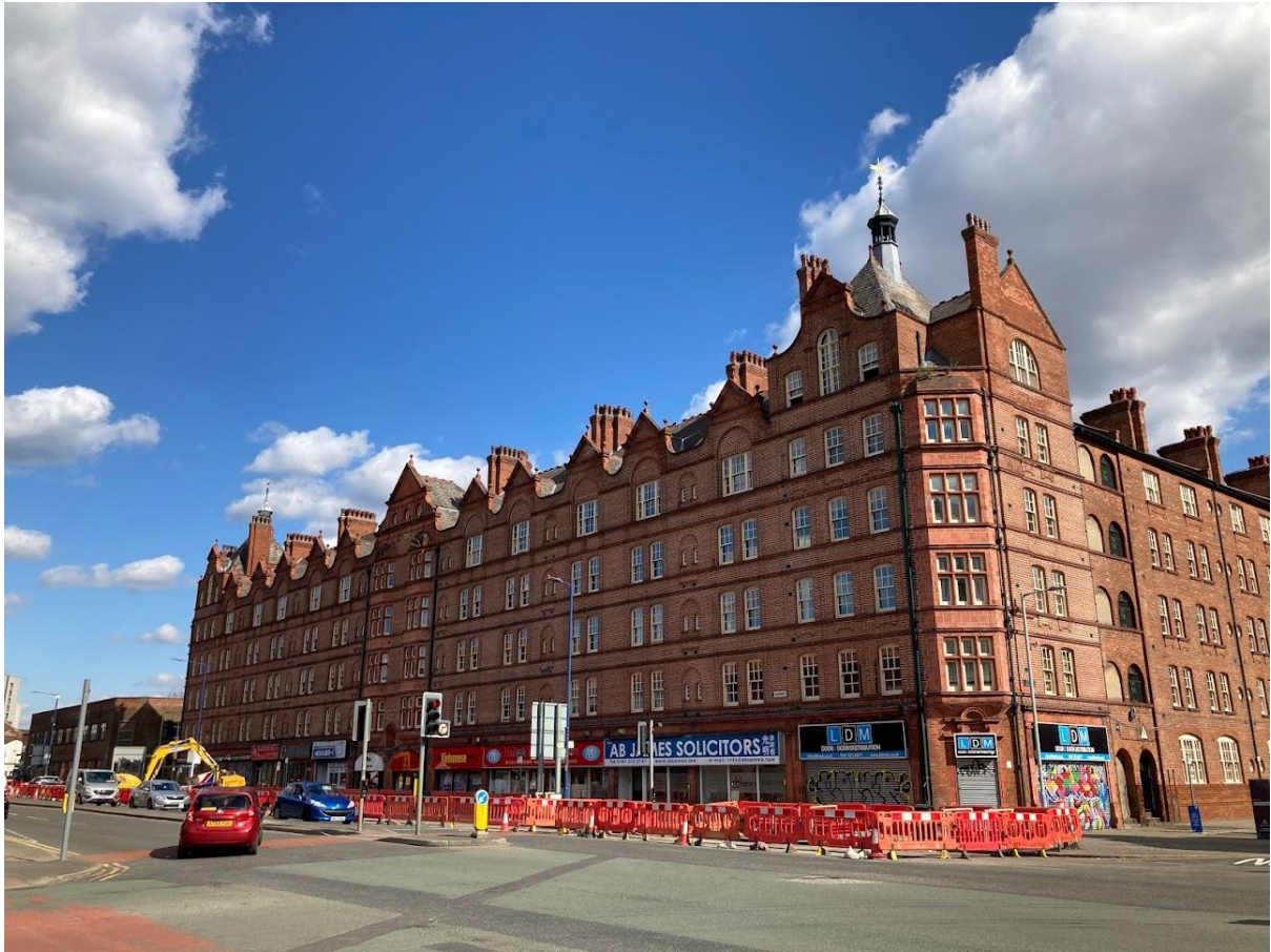
FIGURE 13 – OLDHAM ROAD EXTERNAL ELEVATION
