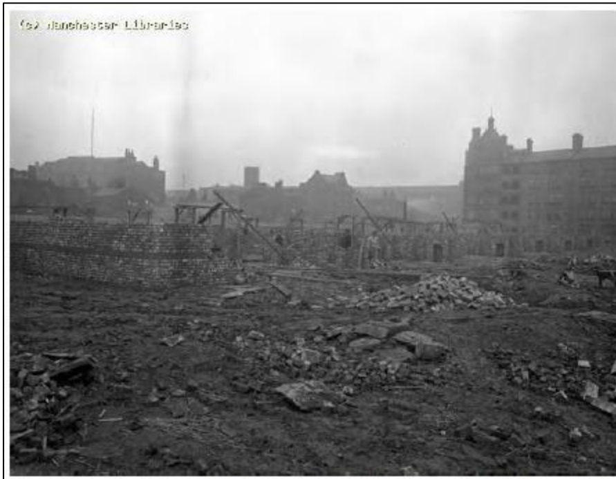
FIGURE 3 - CLEARANCE AND NEW WORKS FOLLOWING COMPLETION OF VICTORIA SQUARE 1898
