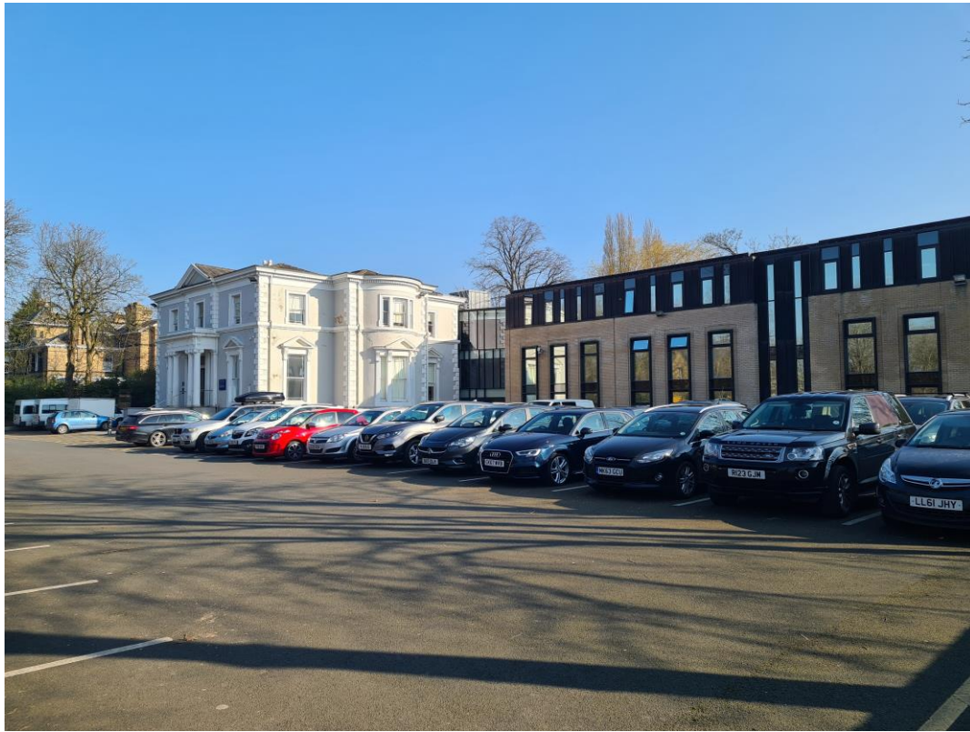
Figure 1: Ward Hall with classroom extension
