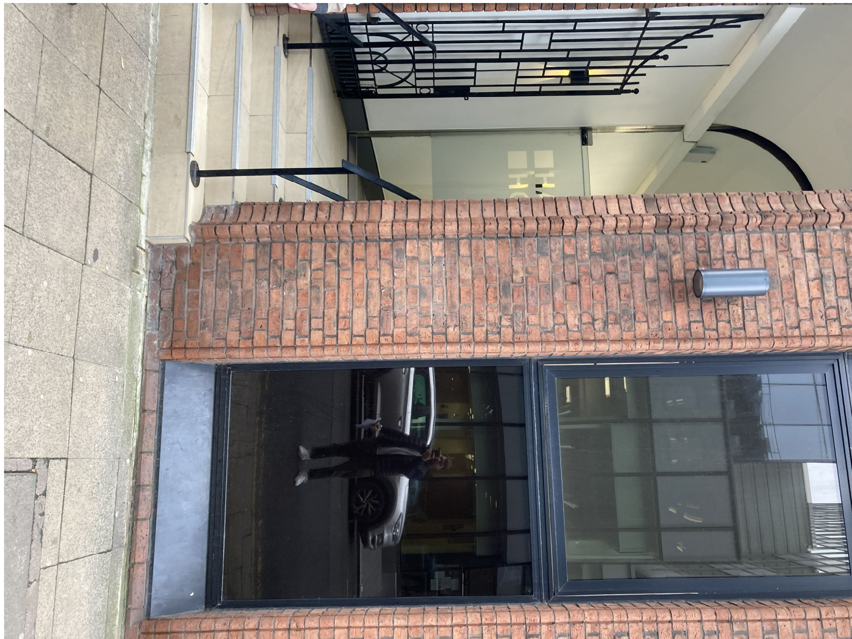
Site Photographs Exterior
