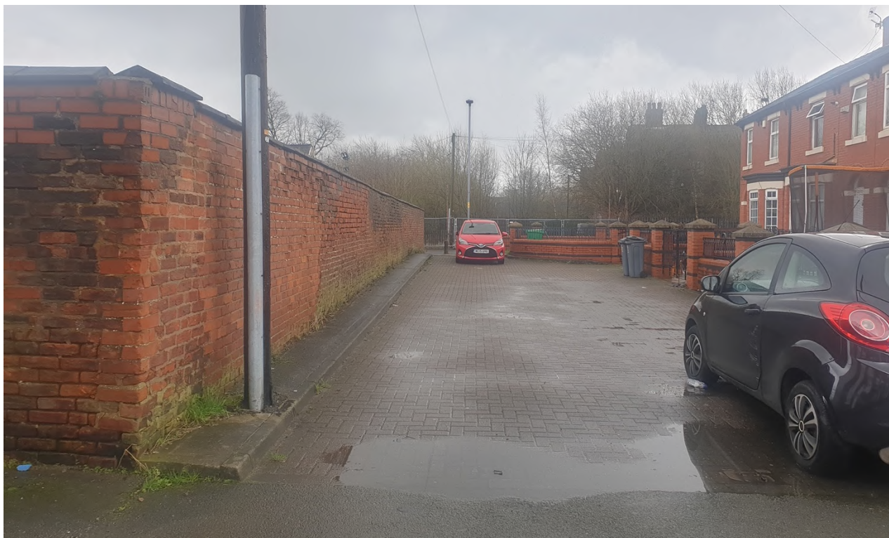
Photograph 2.6 : Unadopted Section of Backwell Street
