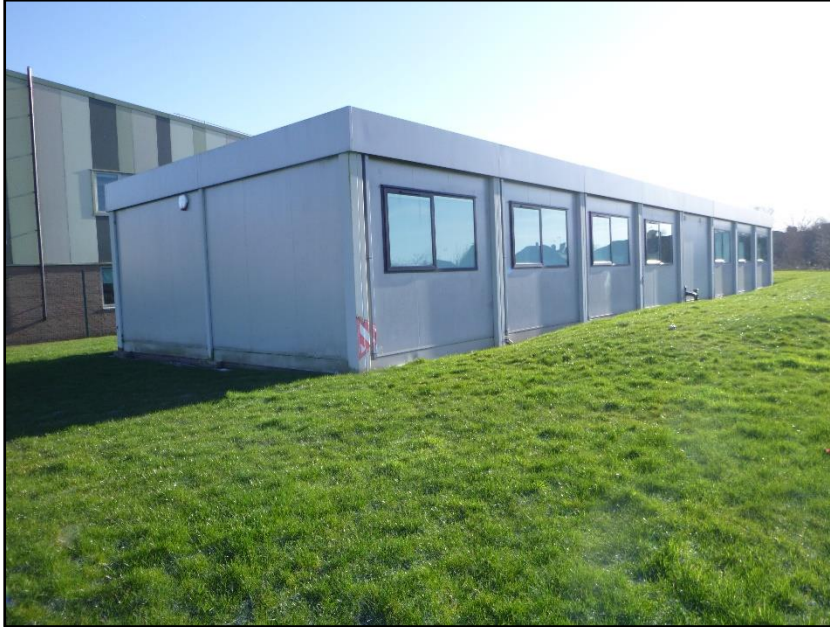
Photograph 5 showing the prefabricated classroom on site
