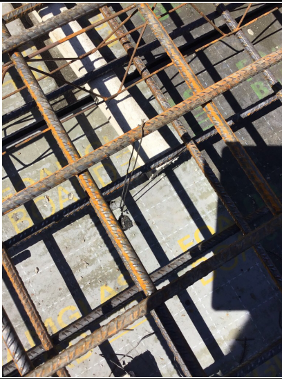
Wire ties holding the membrane to the rebar.
