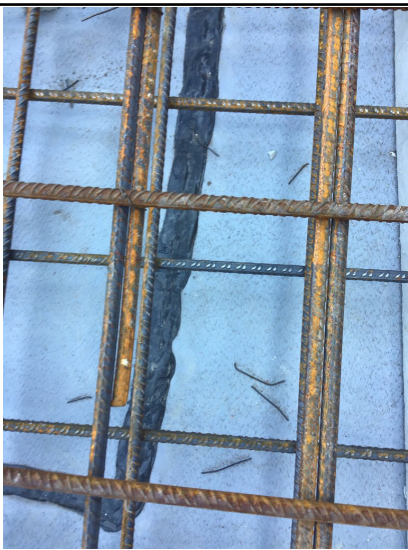
Extrusion weld on Visqueen
