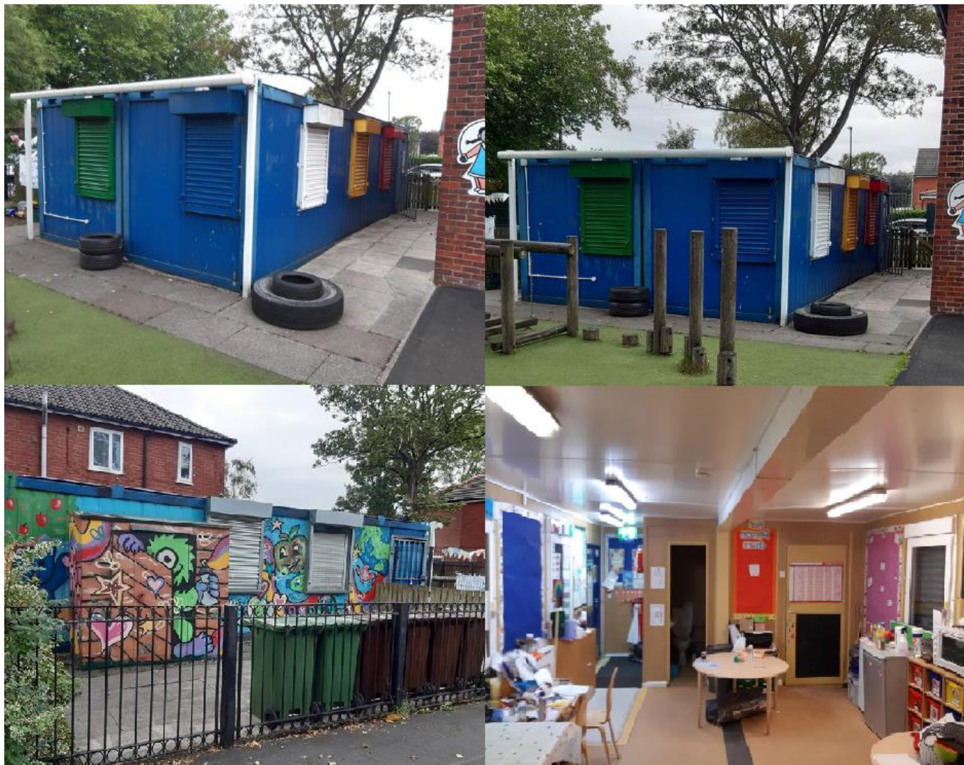
Photograph 1 Medley of photographs showing the external and internal condition of the cabin.
