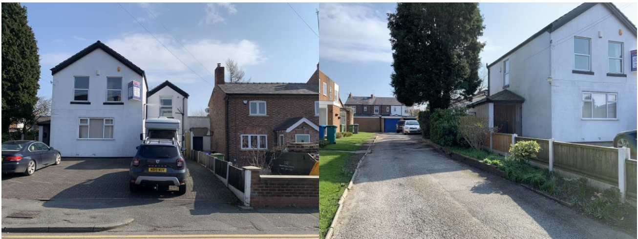
Photograph 1 and 2; Application Site as viewed from Moor End (public highway). Source: Officer's Site Photographs (08.03.2022)
