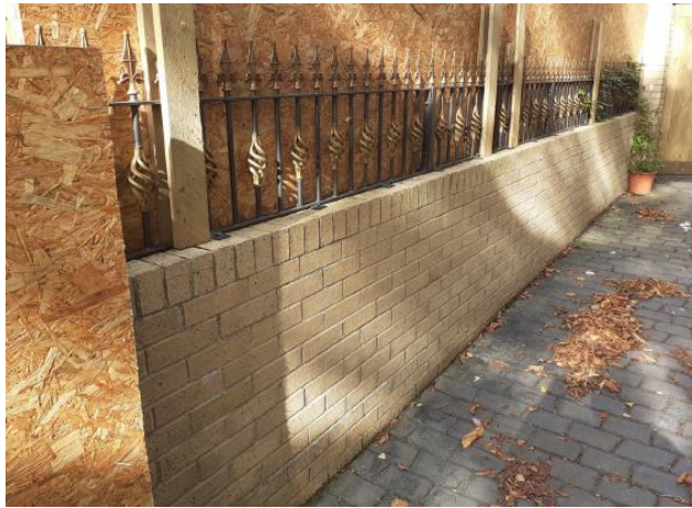
Existing eastern boundary wall
