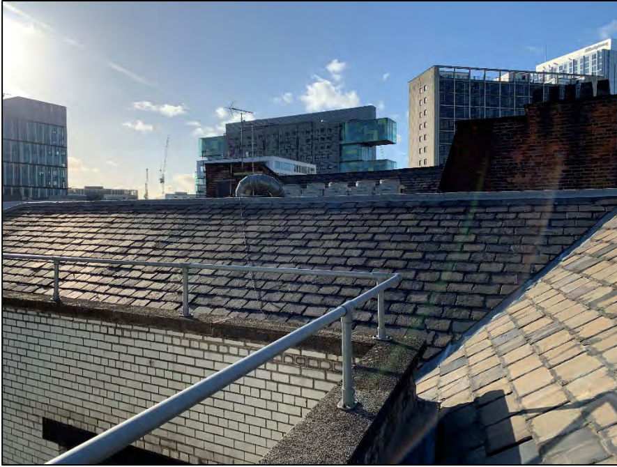
Photograph A2.3: Western rooftop area of site.
