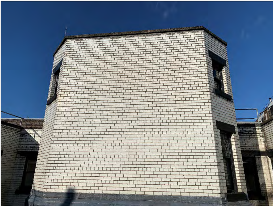
Photograph A2.2: Central rooftop area of site.
