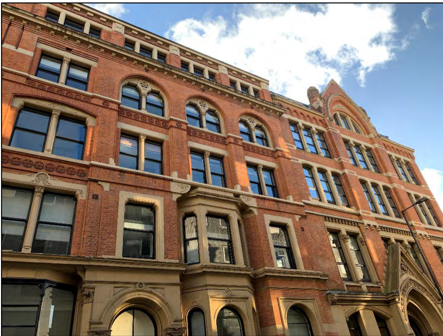
Photograph A2.8: External north aspect of building.
