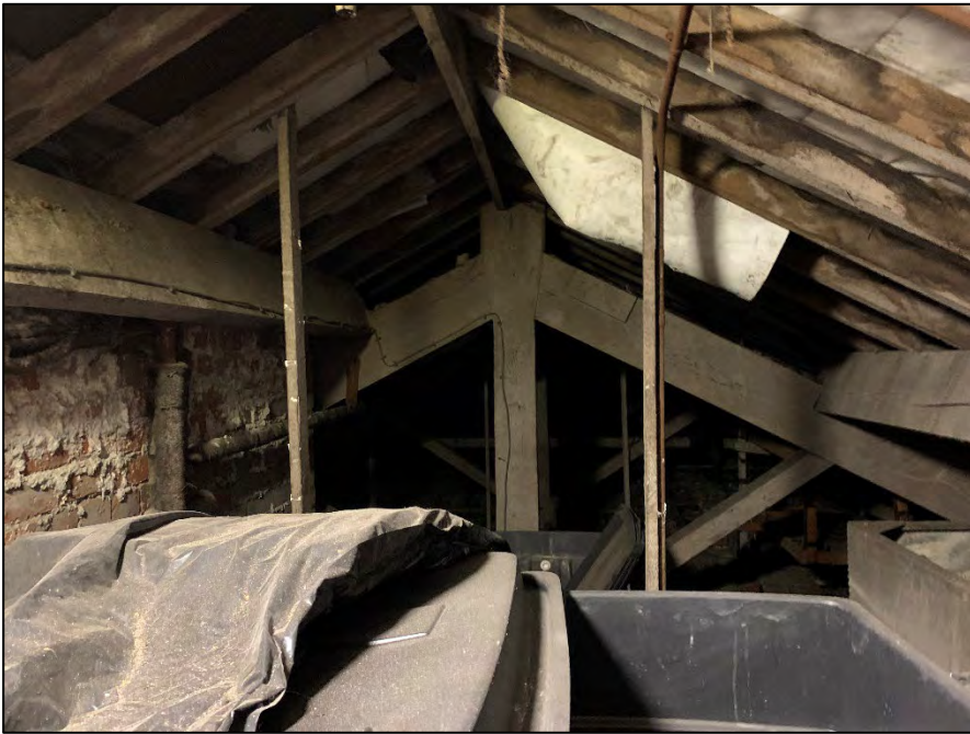
Photograph A2.6: Internal roof void.
