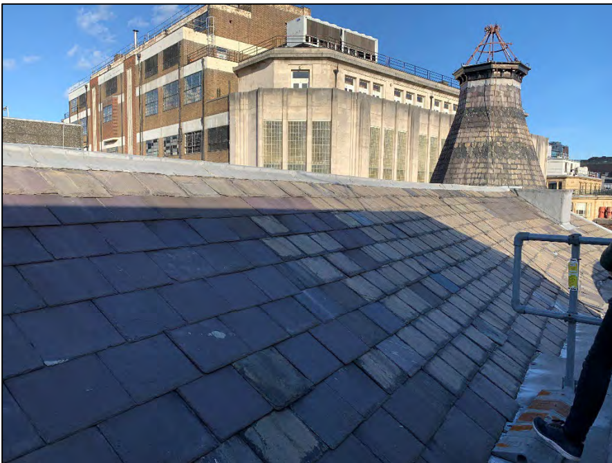
Photograph A2.4: Eastern rooftop area of site
