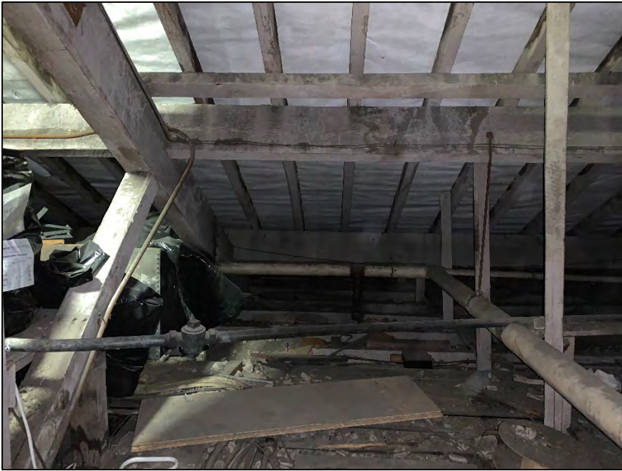
Photograph A2.7: Internal roof void and ceiling lining
