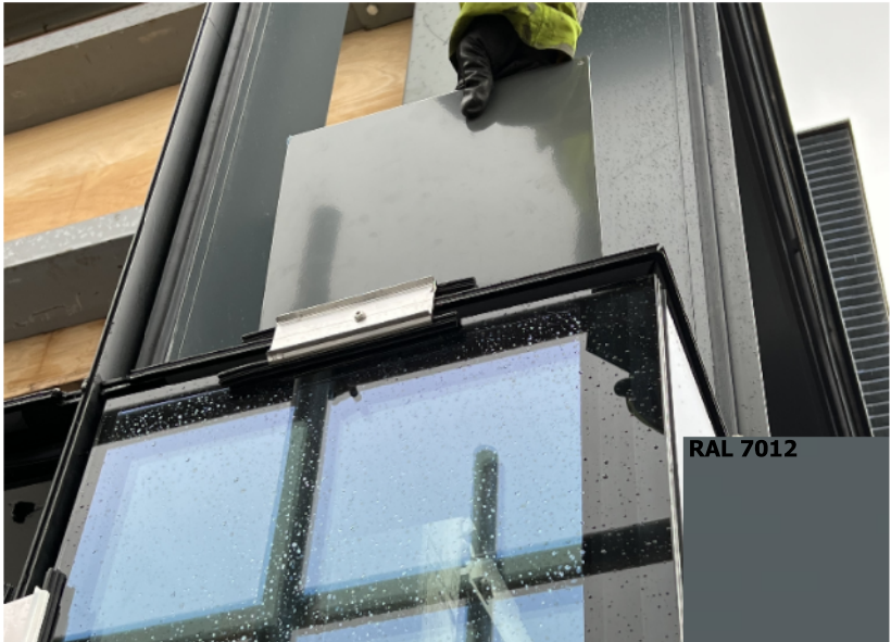
Photograph of 7012 gloss panel at the head of the lift shaft
