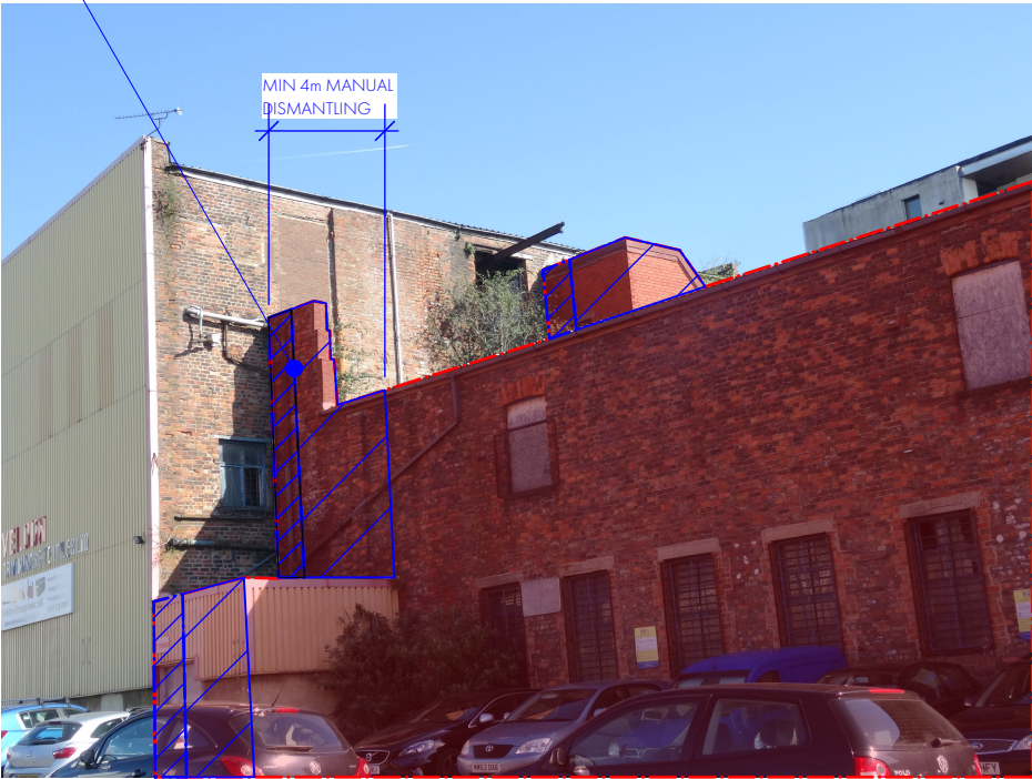
IMAGE 002- PIGEON STREET - Junction between retained and demolished
