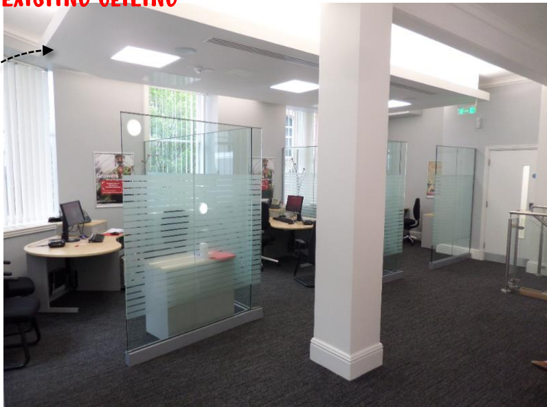
IMAGE SHOWING EXISTING CEILING MADE OF PLASTERBOARD RAFTS
