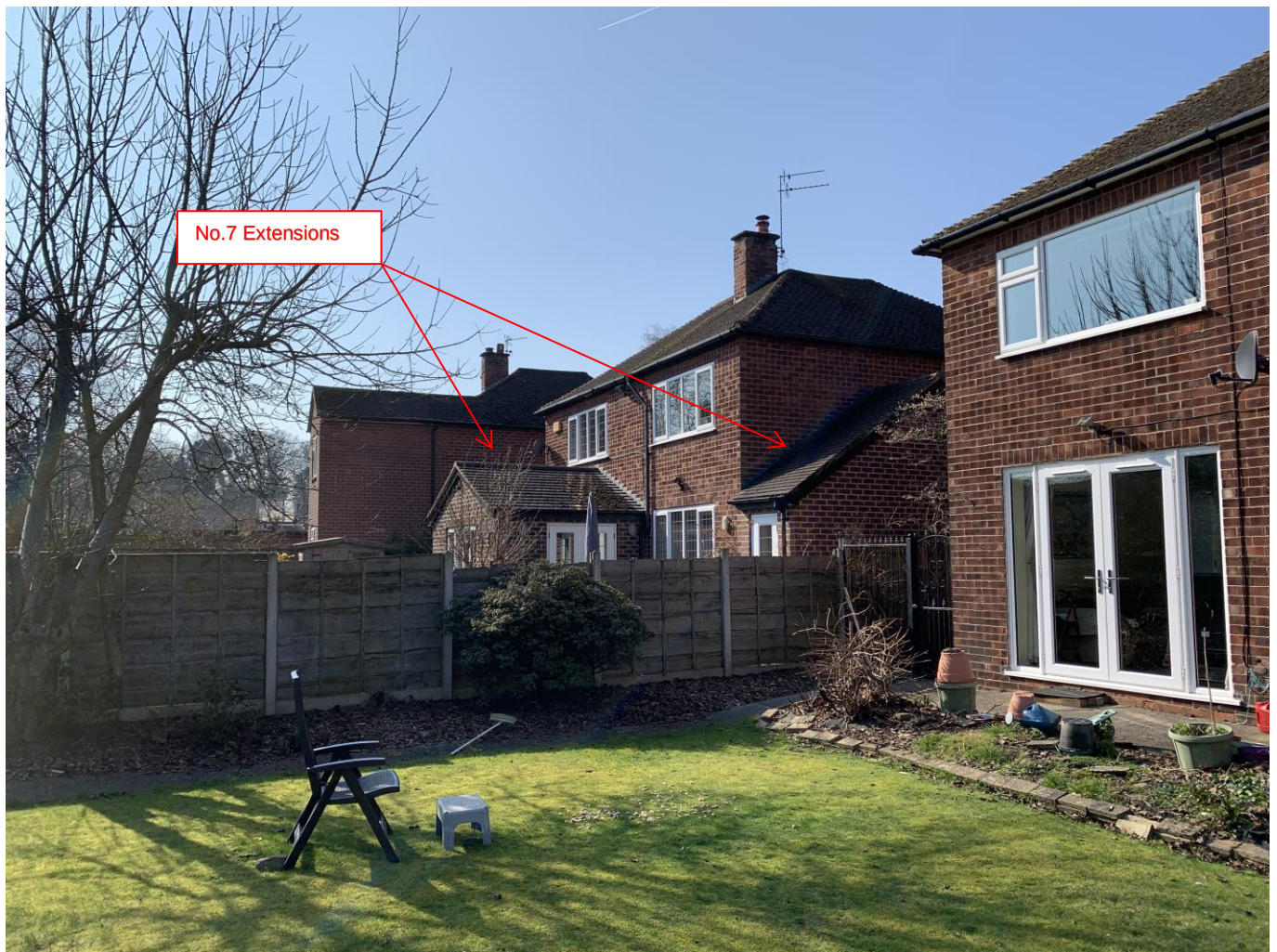
Photograph 2 Rear of 7 Netherwood Road
