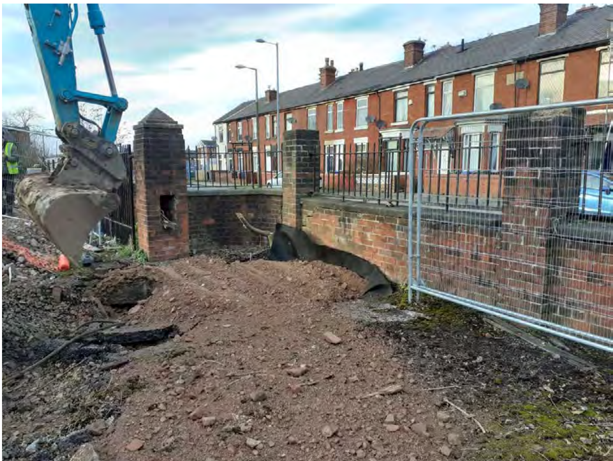
Pic 8 – JK Area 3 with CuTex and backfilled
