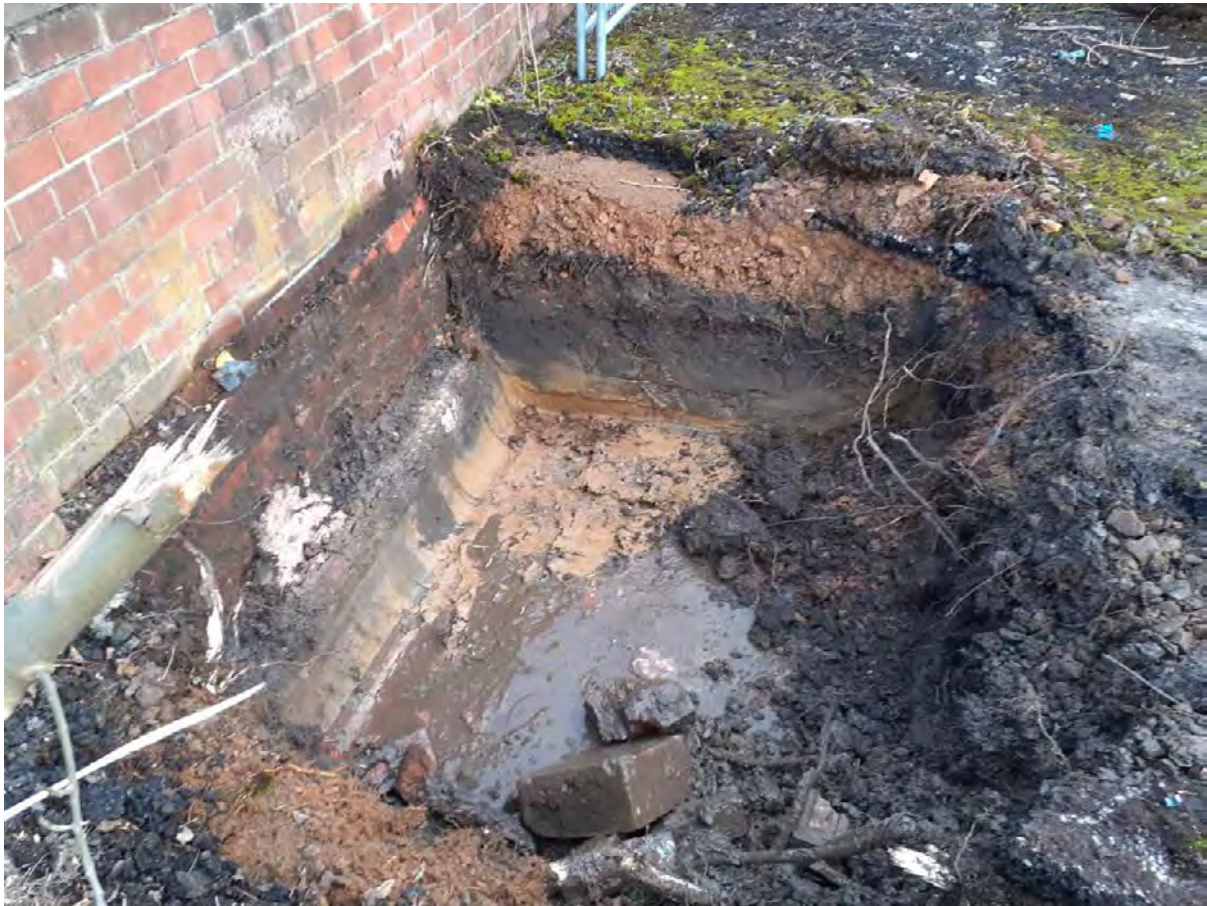
Pic 7 – JK area 3 after excavation
