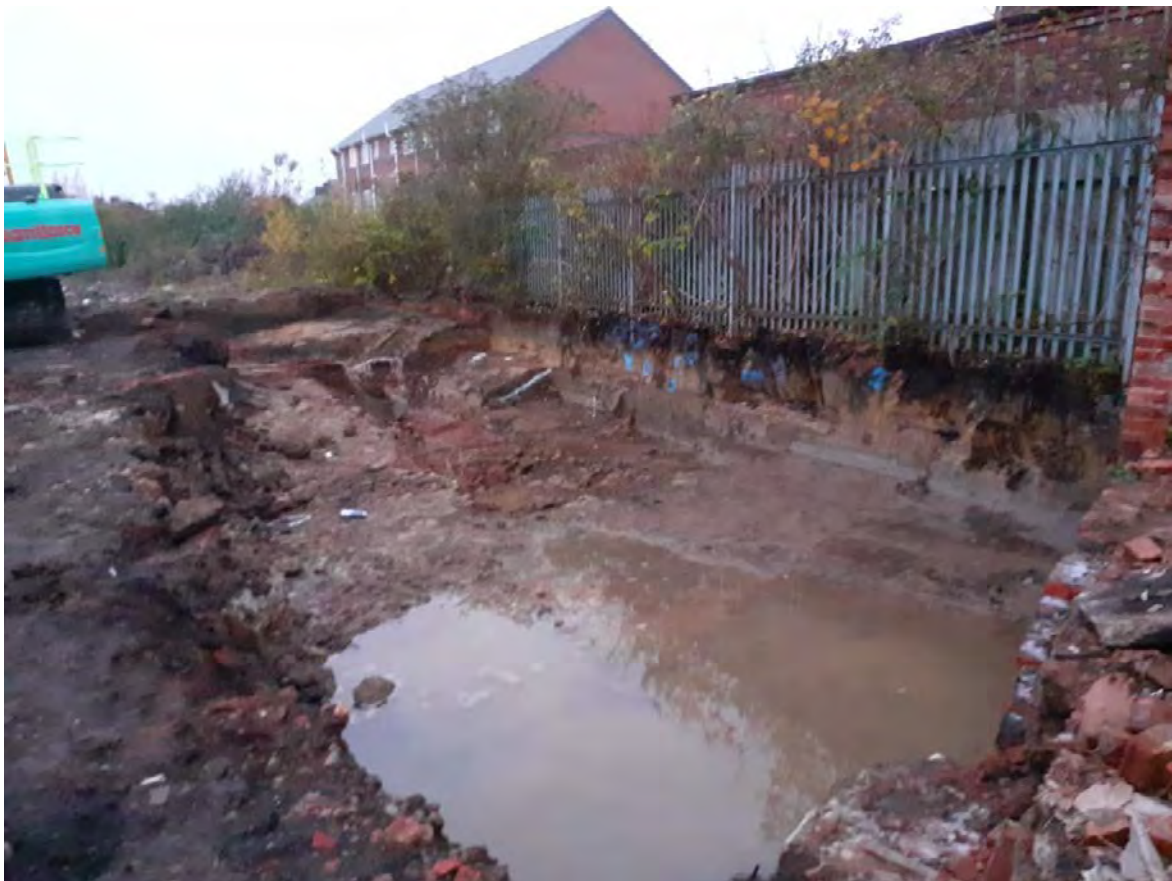
Pic 2 - JK area 1 after excavation
