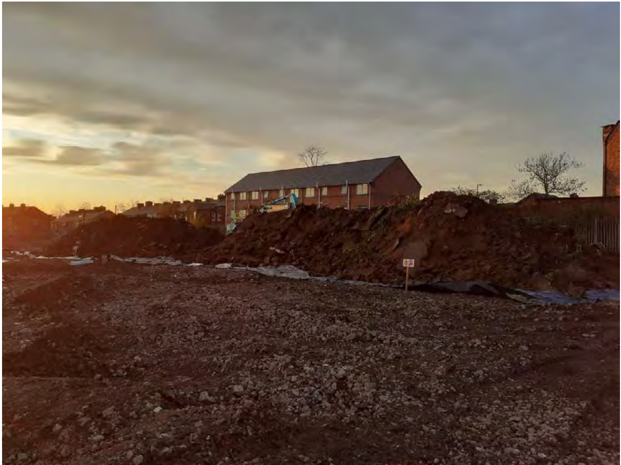
Pic 9 - Final excavated stockpile prior to being moved
