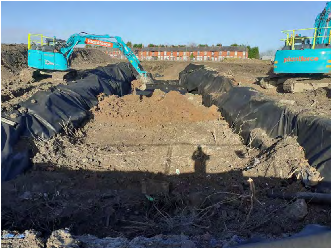
Pic 12 – Cell being filled with JK material
