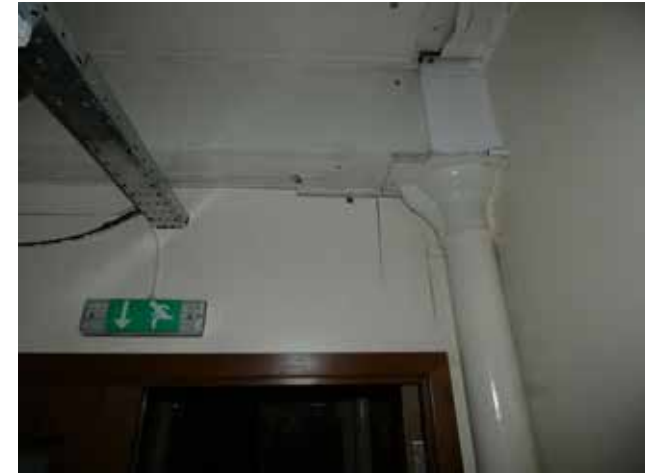
3.33 B028 Typical cast iron column and overlaid beam (Insall)
