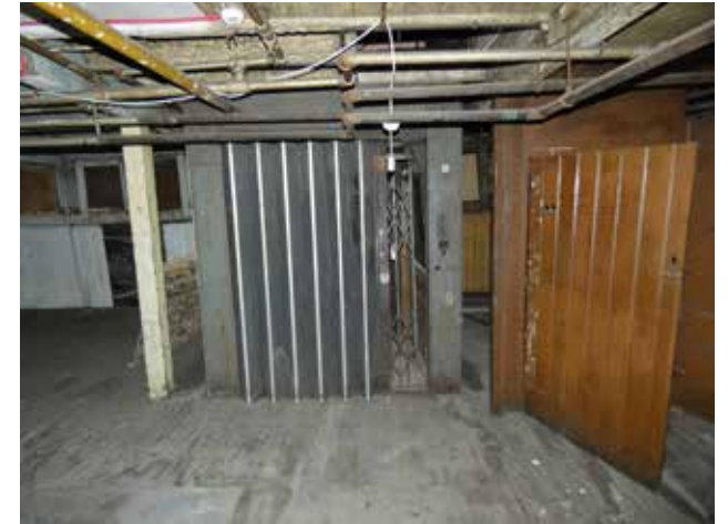
3.96 Lift shaft, FF05
