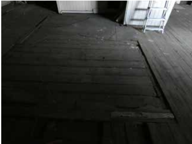
3.92 Floor with potential infilled hoist, FF004
