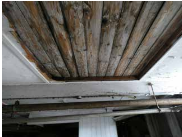
3.95 Timber boarding to ceiling, FF005
