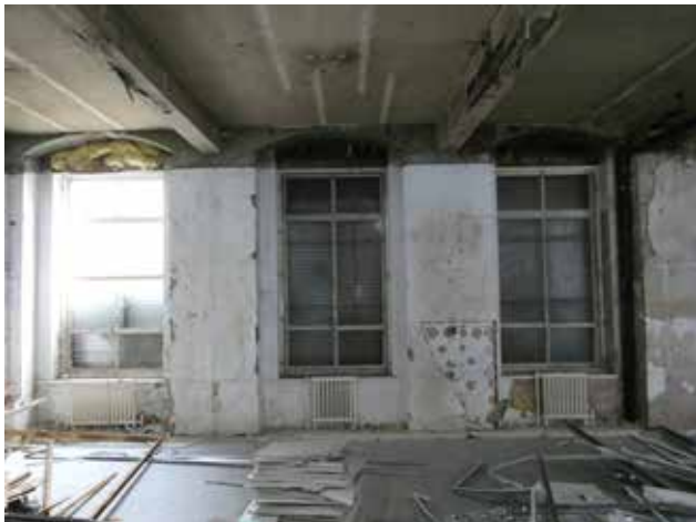
3.40 Arched lintels in rear wall, Ground Floor
