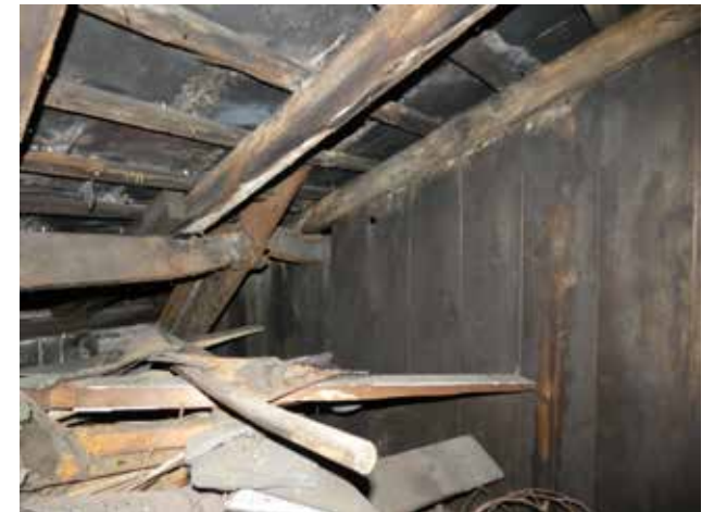
3.105 View of eaves, with cast iron rafters and purlins
