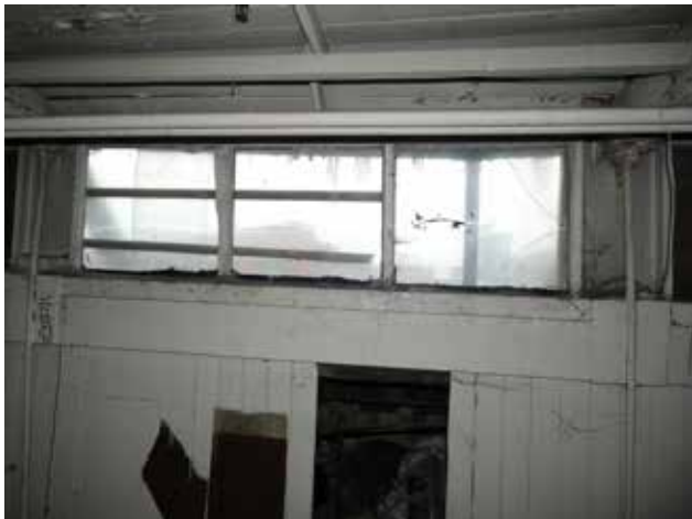
3.93 Modern reeded glazing, FF004
