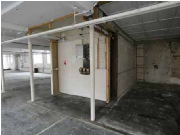
3.44 Partitions around timber staircase, First Floor
