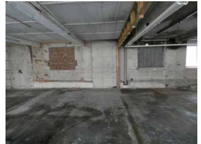
3.48 Rear wall, First Floor
