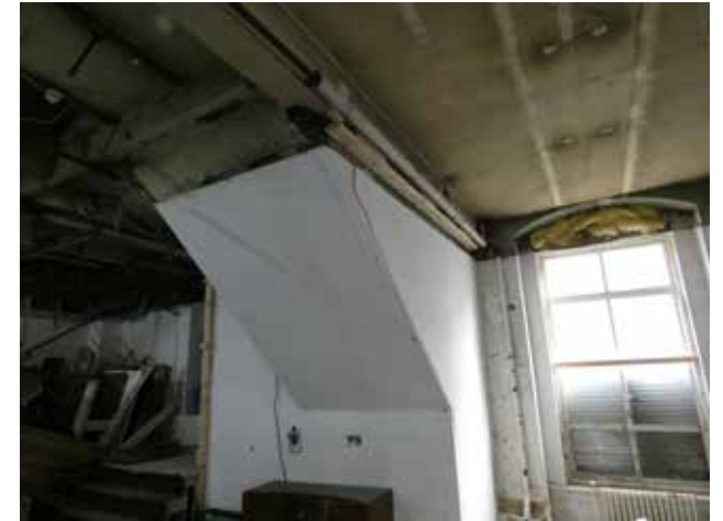
3.42 Plasterboard around timber staircase, Ground Floor
